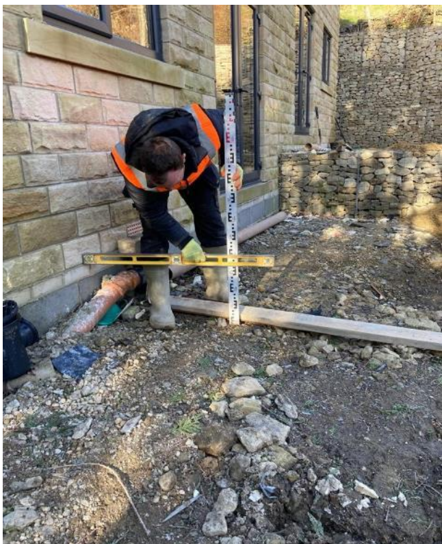
Preparation prior to placing aggregate and hard paving to the rear, with sub base shown to be 300+ mm below finished ground level.
