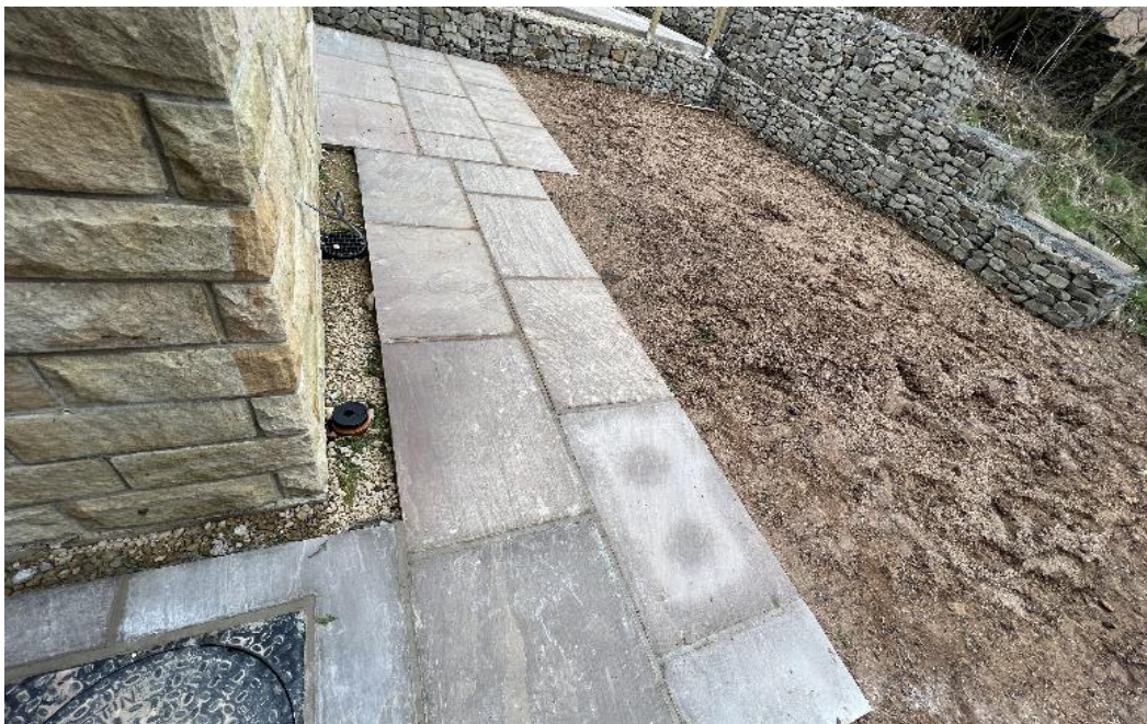
Finished hard paving to the rear.
