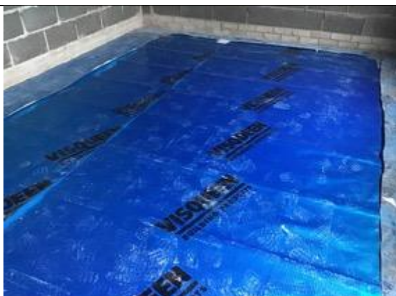
Plot 7 infill installation
