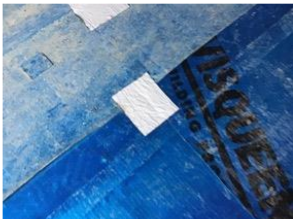
Plot 7 T joint SAGM patch
