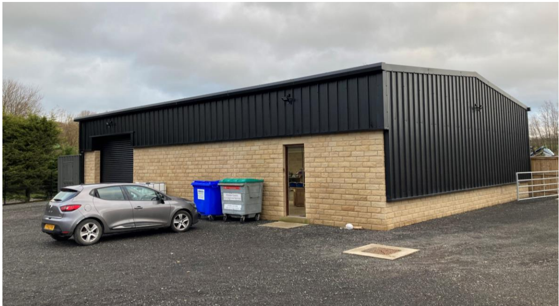
Figure 4: The workshop building as constructed (looking north-east)
