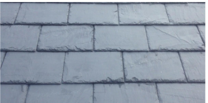
Coursed reclaimed yorkshire gritstone walls coined to match neighbouring properties & natural slate tiles to all plots
