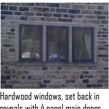
Coursed reclaimed yorkshire gritstone walls coined to match neighbouring properties & natural slate tiles to all plots
