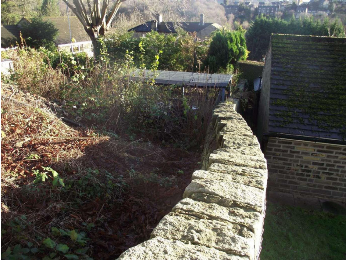
Photo 2 – Lateral distortion and bow to head of wall in vicinity of mature broad leaf tree.
