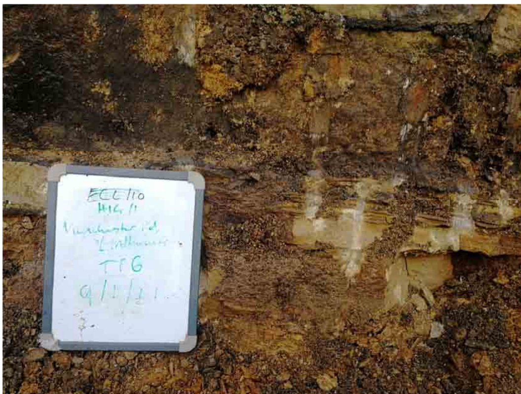
Photograph 4: Close-up of exposed foundation in TP6
