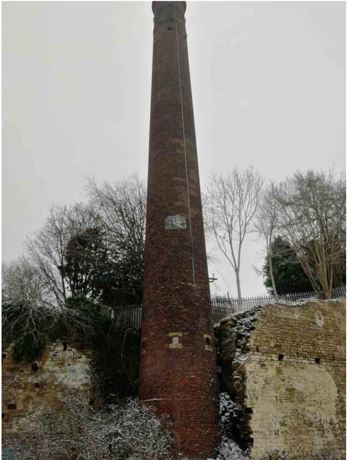
Photograph 13: Chimney at northern end of Area A.
