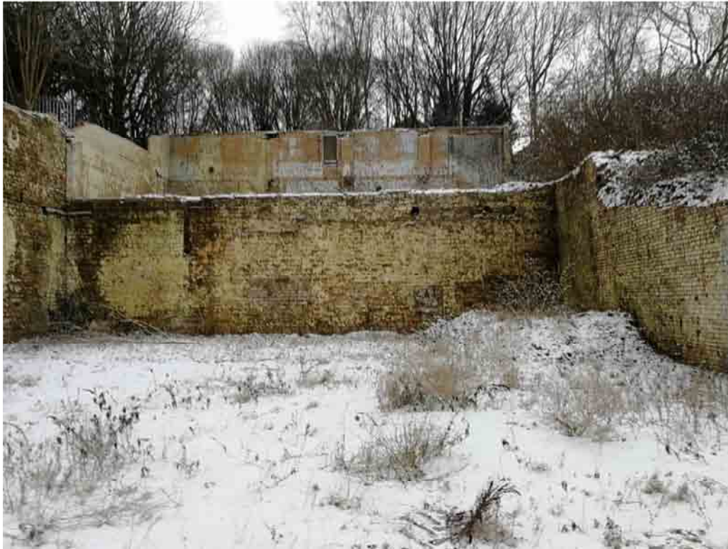
Photograph 1: Sandstone retaining wall in background, brick retaining wall to the right. Photograph facing south.
