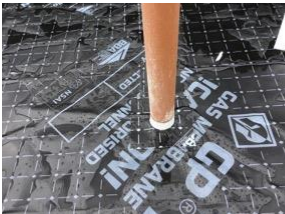
Plot 7 pipe penetration sealed using preformed top hat and SAGM
