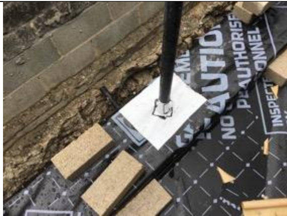
Plot 8 service pipe seal using SAGM
