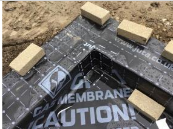
Plot 7 corner detail using preformed corners
