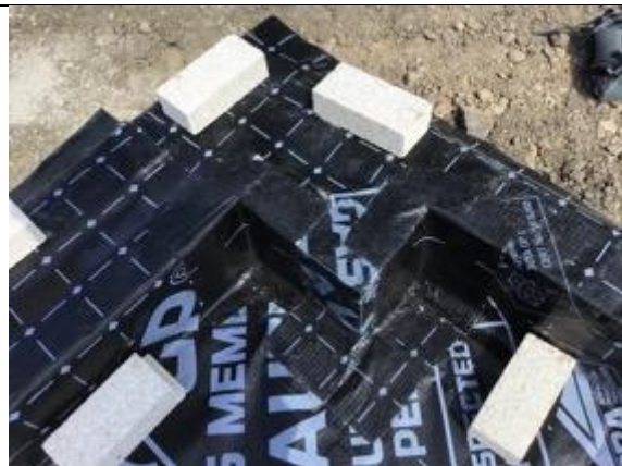
Plot 10 corner detail using preformed corners
