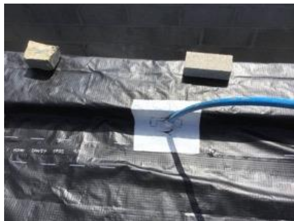
Plot 10 corner detail using preformed corners
