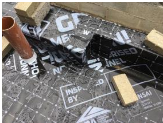
Plot 8p pipe penetration sealed using preformed top hat and SAGM and door threshold using preformed corners
