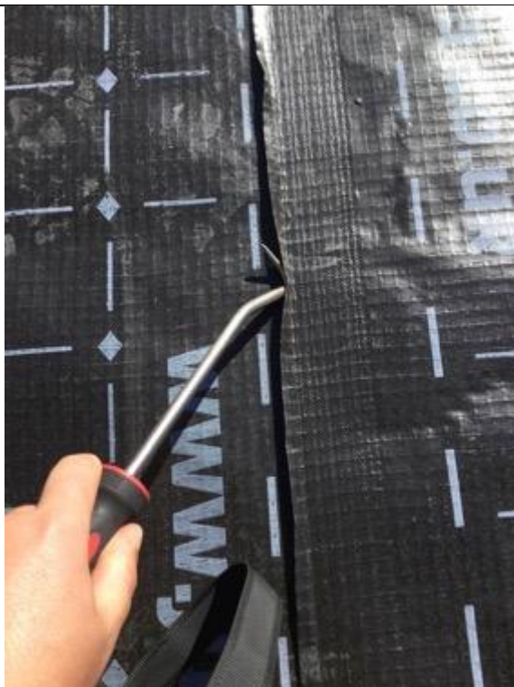
Pick probe testing carried out to the mechanical weld joint.
