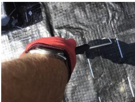
Plot 11 hand welded joint being pick tested
