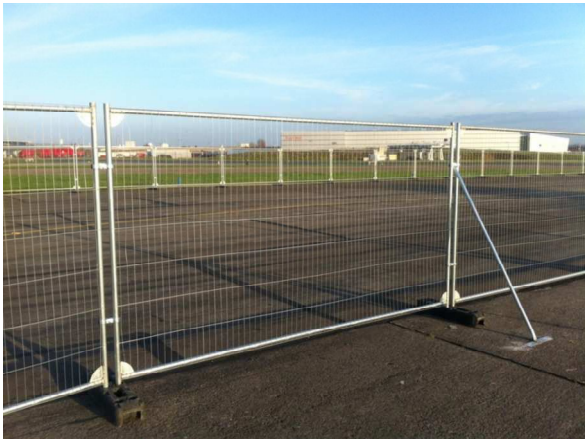
Inset 2: 'Heras' Tree Protection Fencing
