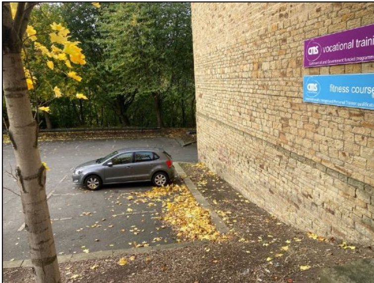
General view to the south west looking at car park at rear
