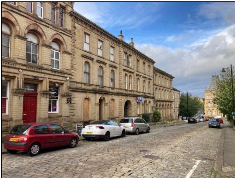
General view to the west looking at site from Station Road
