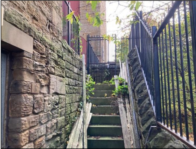
View of steps at rear of site
