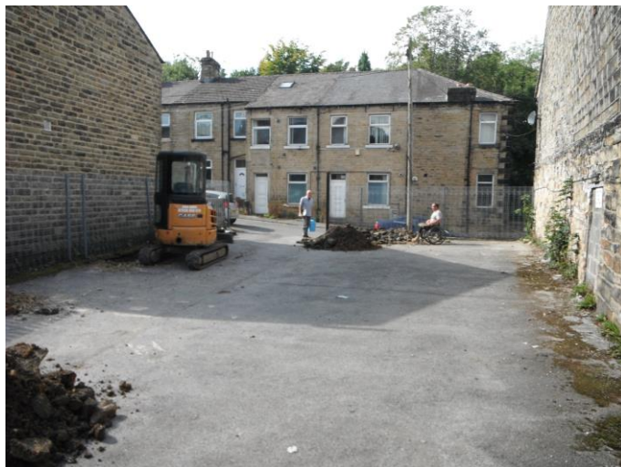
Figure 3 – View to Commercial Street.
