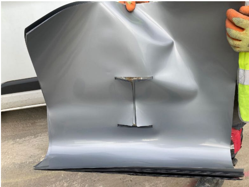
Plate 2: Pre-cut gas membrane sections for around steel columns (11/08/2021)
