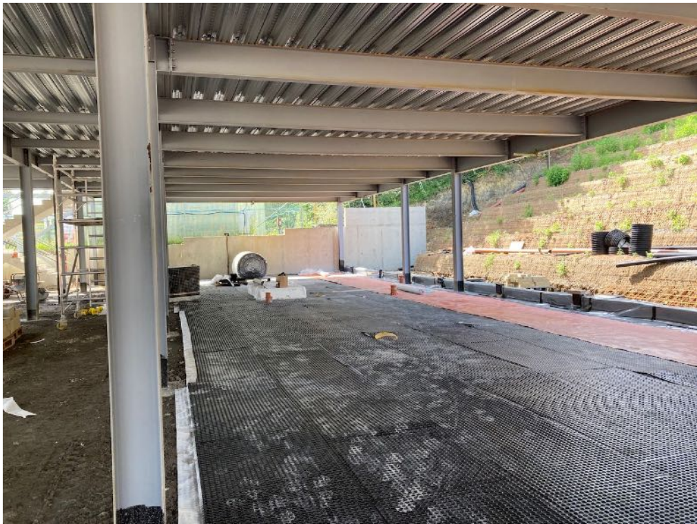
Plate 8: Void former installed across north half of building (13/08/2021)
