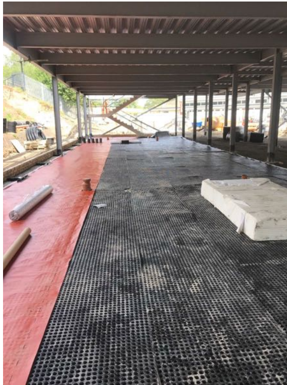
Plate 5: Beginning installation of gas resistant membrane (12/08/2021)
