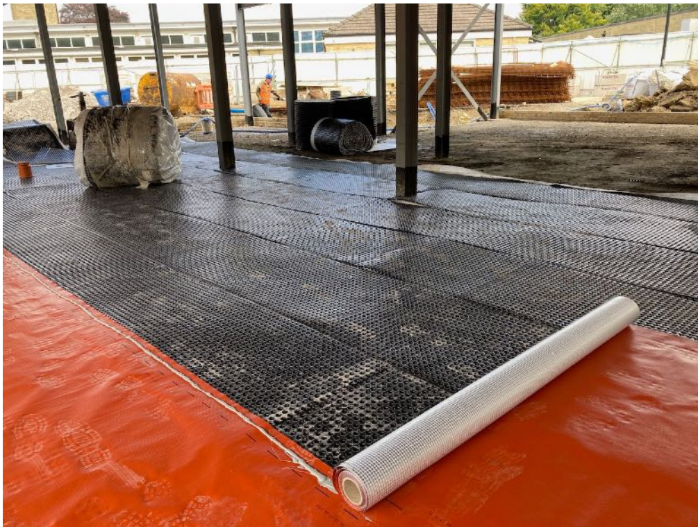
Plate 16: Membrane rolled out over butyl sealant (16/08/2021)
