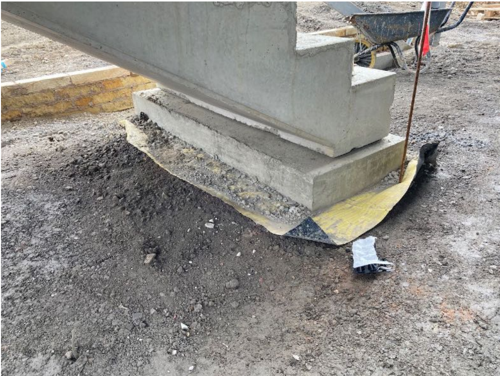
Plate 3: Section of gas membrane laid beneath internal concrete steps (11/08/2021)
