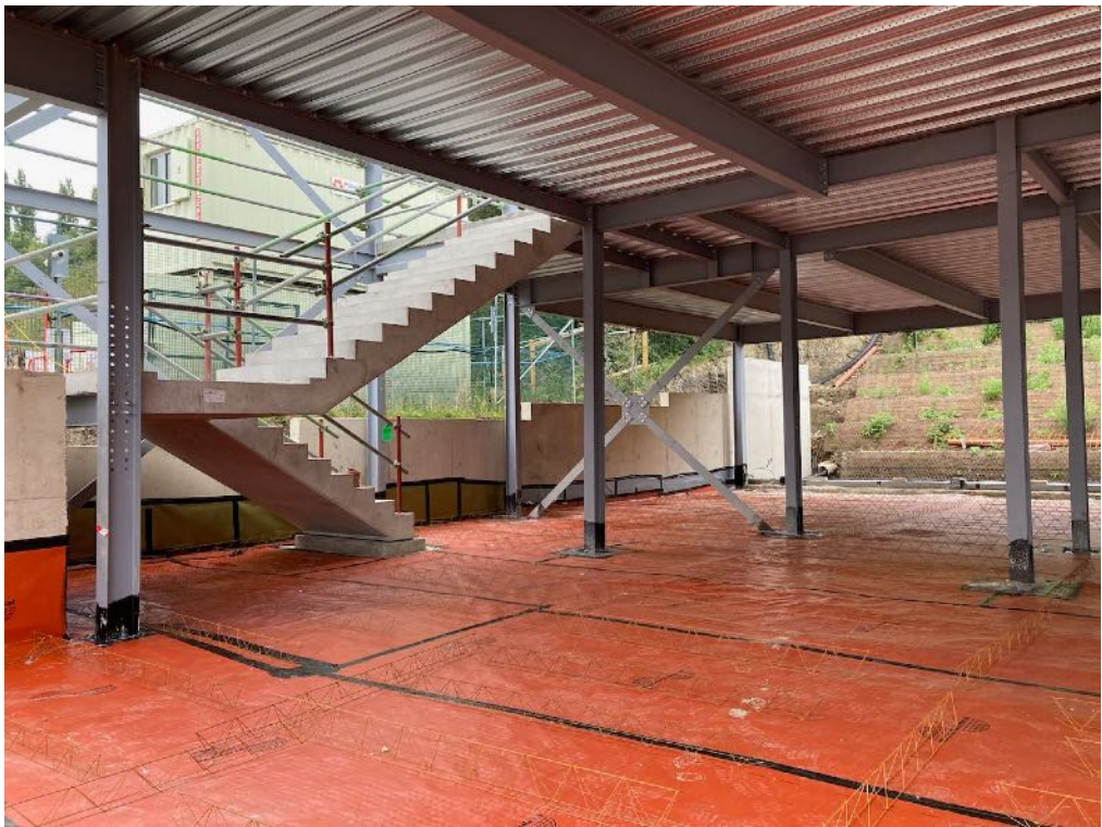
Plate 23: Risers for mesh reinforcement placed over membrane (01/09/2021)
