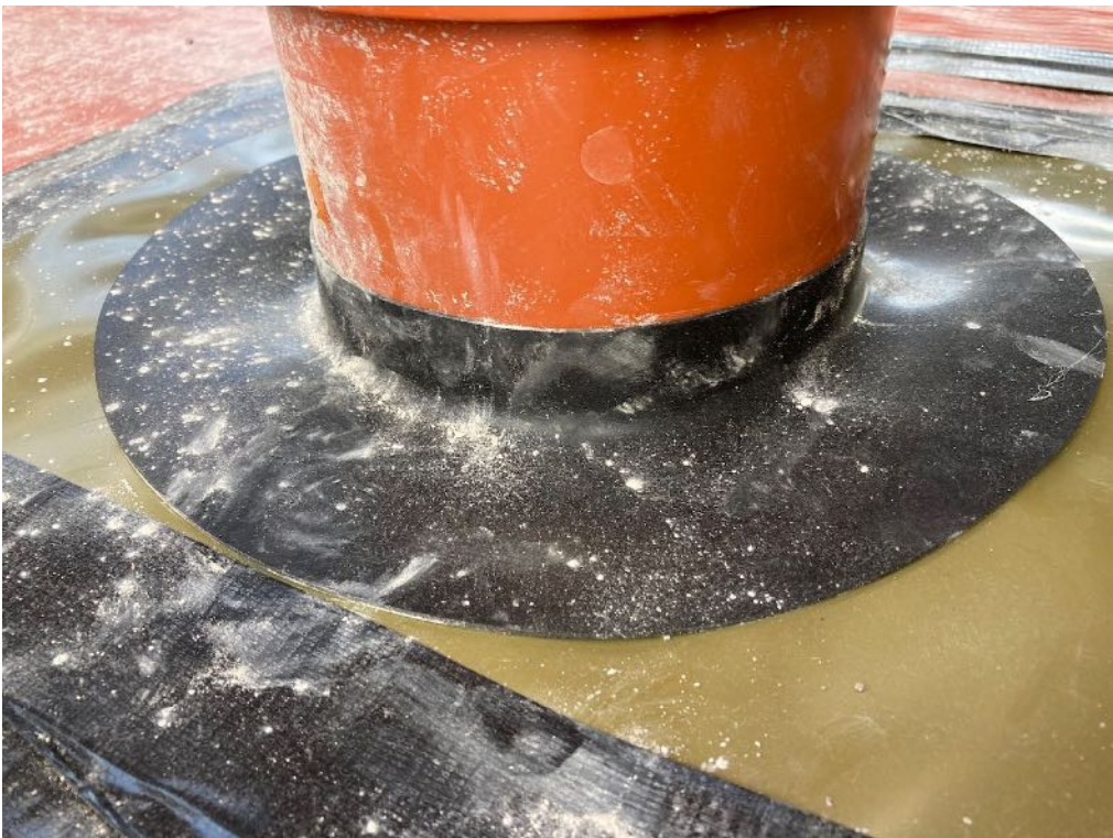
Plate 13: Service entry following rubber top hat & sealing (13/08/2021)
