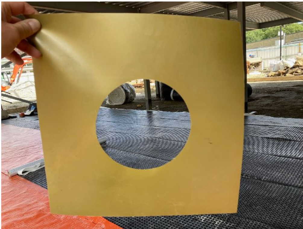
Plate 12: Example of pre-cut gas membrane placed over service entries (13/08/2021)
