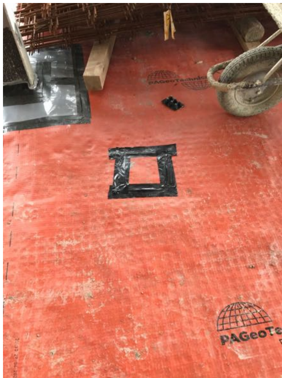
Plate 20: Local repair of gas membrane where scratched by mesh (26/08/2021)
