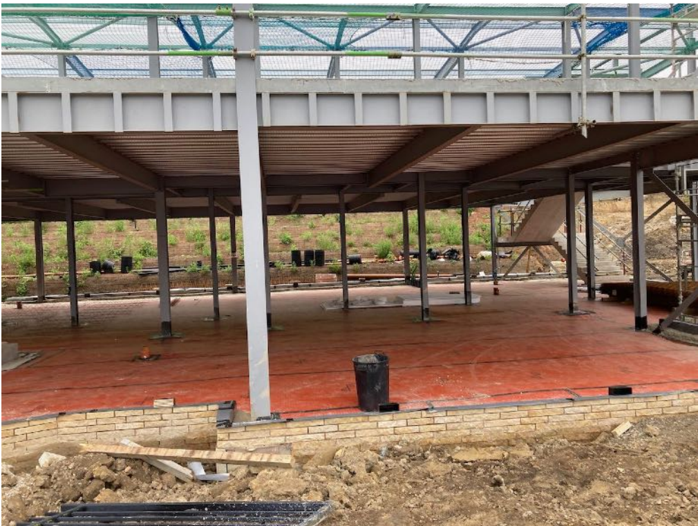
Plate 21: Membrane placed across whole footprint area (01/09/2021)
