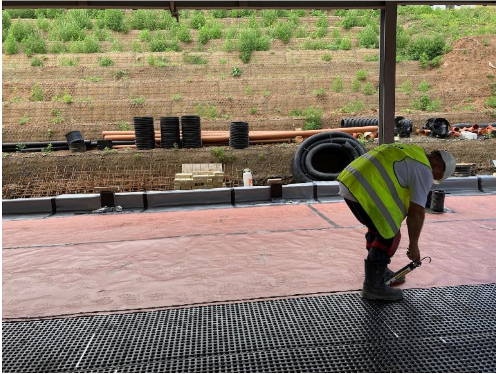
Plate 15: Reinforced Butyl sealant being applied along membrane joints (16/08/2021)
