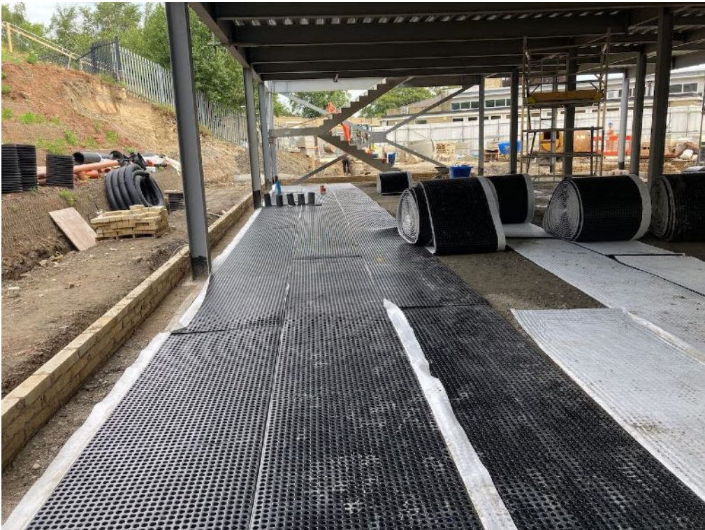
Plate 4: First three rows of void former laid (11/08/2021)
