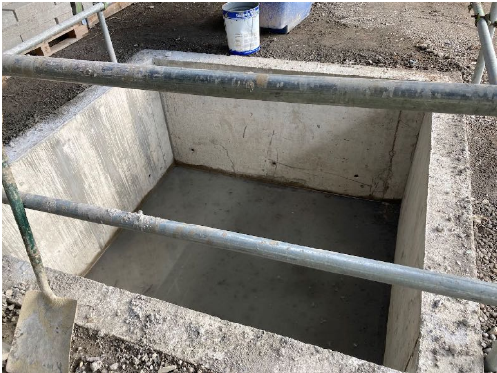
Plate 1: Lift shaft formed (11/08/2021)
