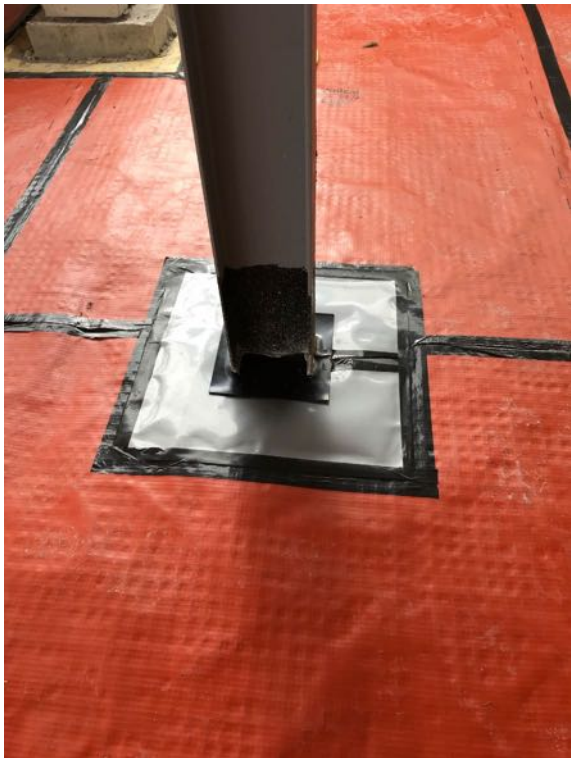
Plate 18: Sealing around internal steel columns (26/08/2021)
