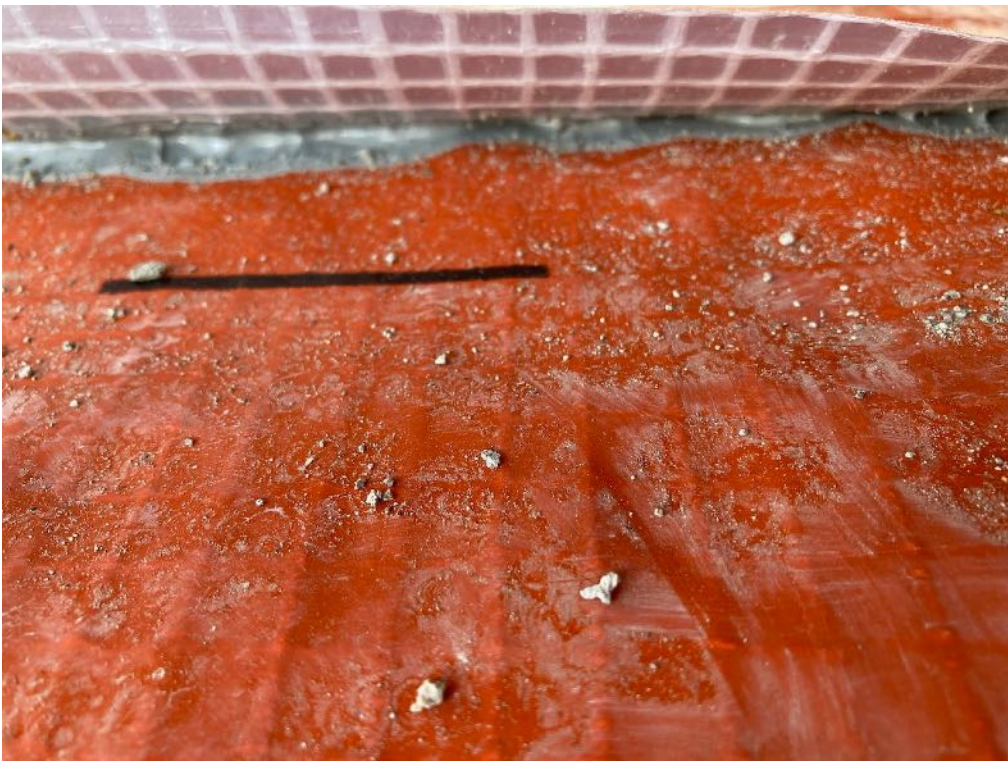
Plate 9: Close-up of joint sealed using SAP Butyl reinforced sealant (13/08/2021)
