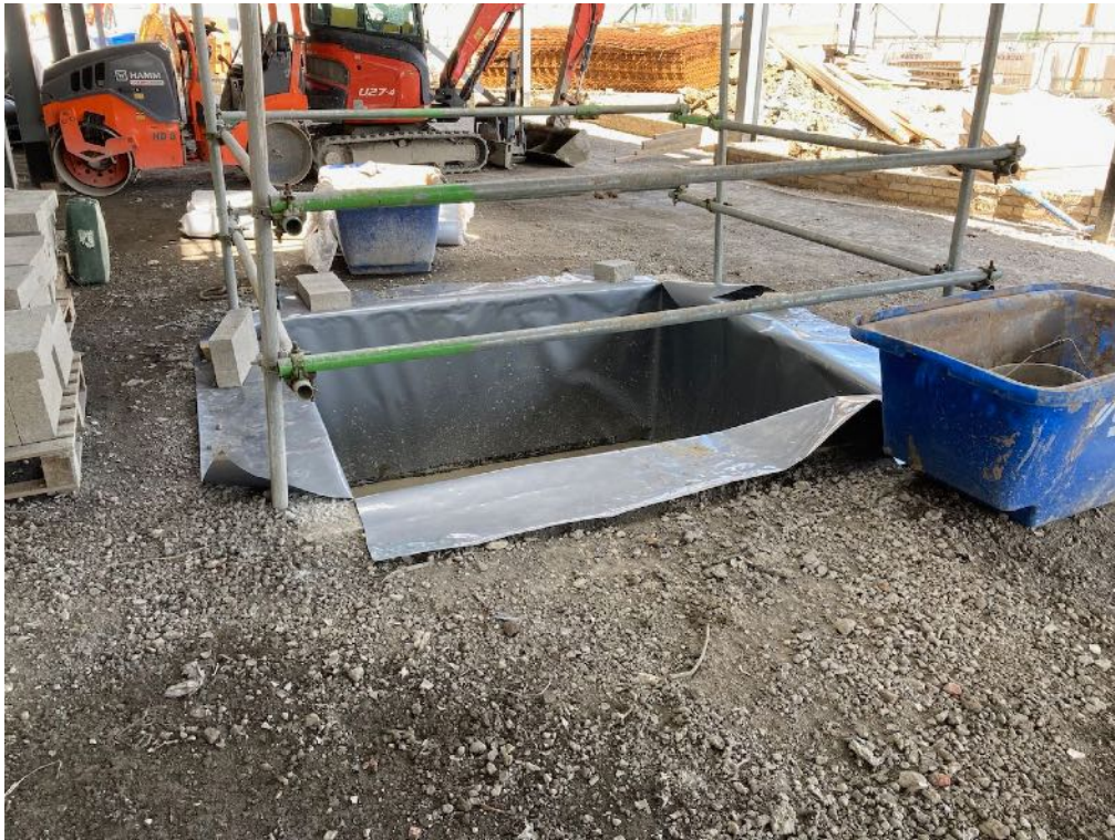
Plate 11: Rhinoplast membrane installed in lift pit & lapped over (13/08/2021)
