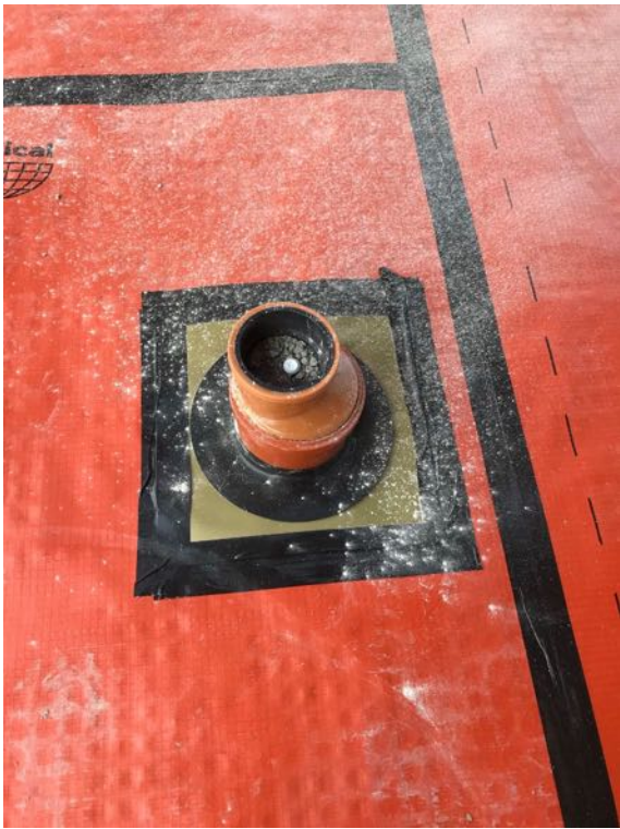
Plate 7: Close-up of service entry sealing (12/08/2021)
