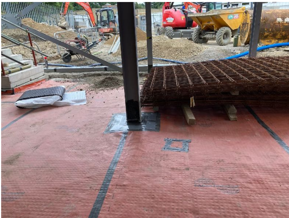
Plate 24: Gas membrane lapped over first step of internal stairs (01/09/2021)
