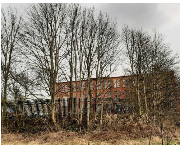
Photo 5: G16, at the eastern boundary
