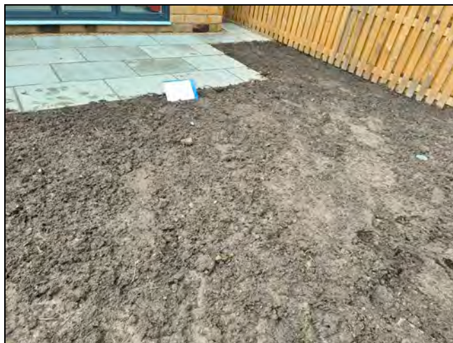
Plot 33 refilled with new clean stockpile and sampled.
