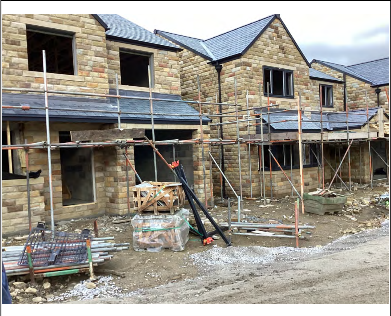
Overview of verified area - Garage Infill
