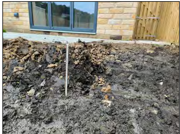
Plot 33 Removal of contaminated topsoil and depth proving(R)
