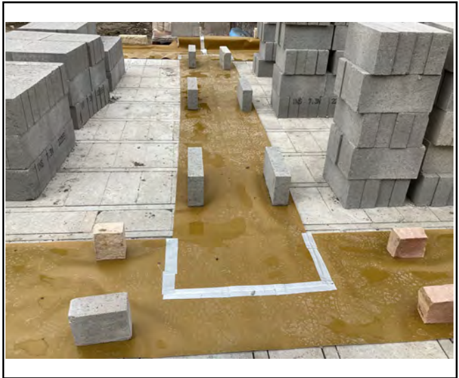
View showing the Visqueen Ultimate
