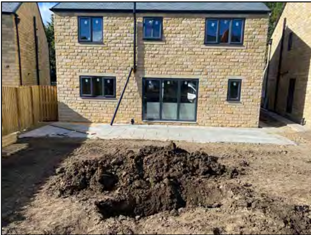
Rear Garden of Plot No 28 showing topsoil proving 600mm depth
