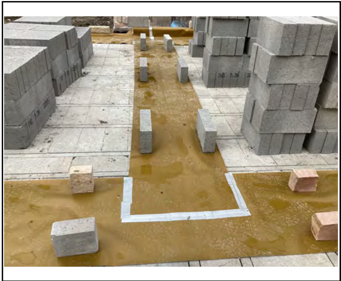
View showing the Visqueen Ultimate
