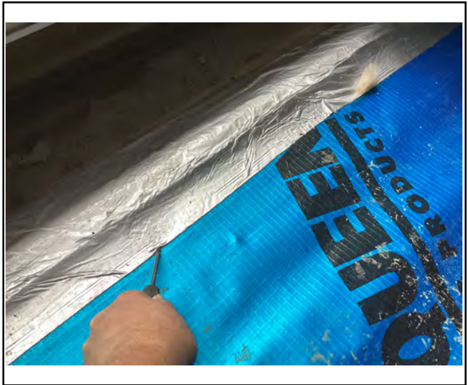
Mechanical Point Stress Test to
