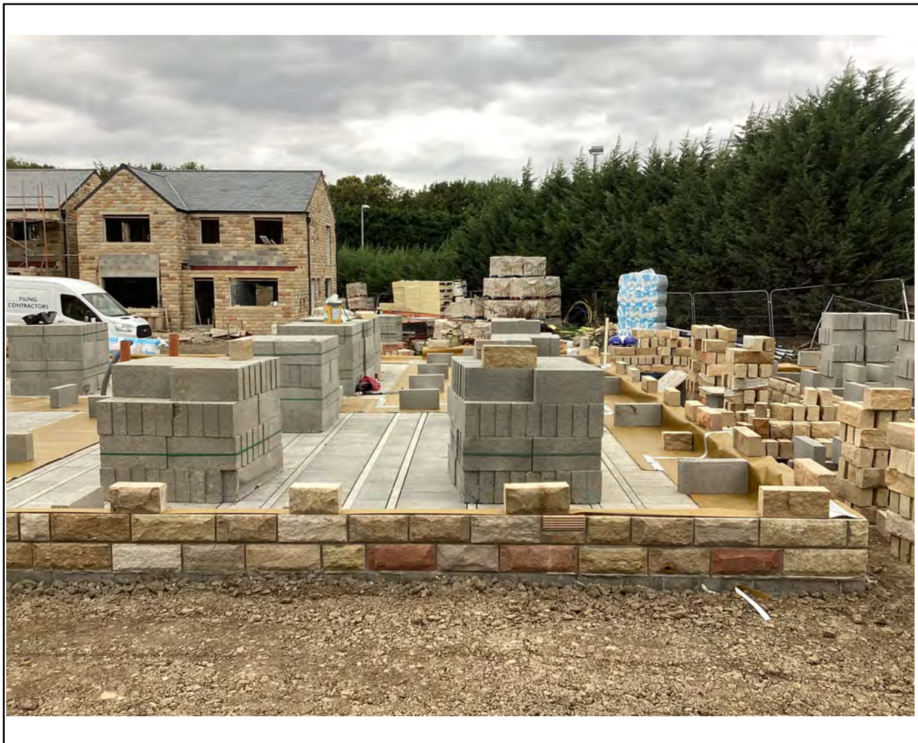
Overview of verified area - perimeter/internal walls
