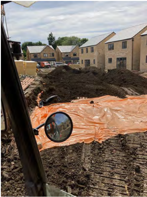
Laying of membrane and topsoil Plots 26 and 27
