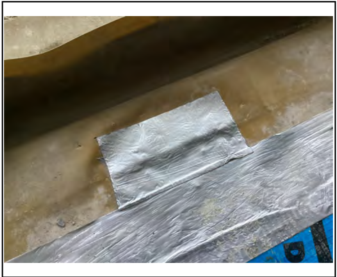
Remediation completed to the
