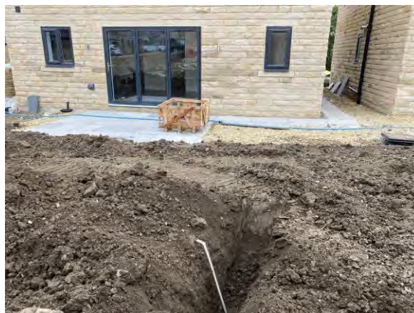
Photos showing the rear gardens of Nos. 22 -25 proving 600mm of topsoil
