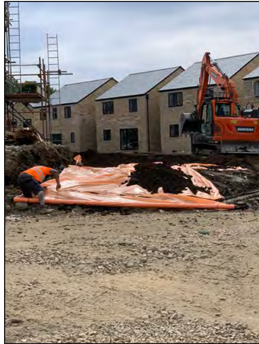
Associated Photos Testing TP depths and Sampling. Laying of membrane prior to topsoil
