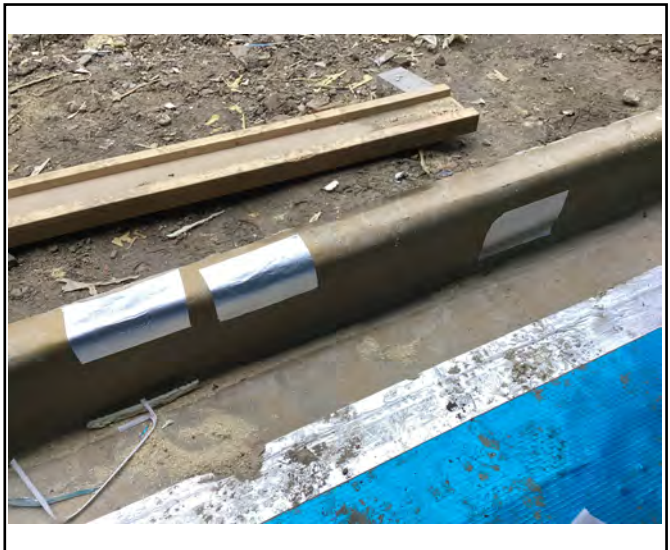
Remediation completed to the
