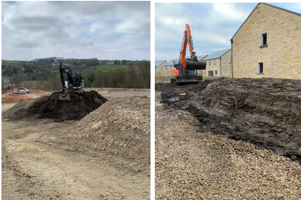
Figure 6 Topsoil stockpiles Hade Edge (left) and Shepley (right)
