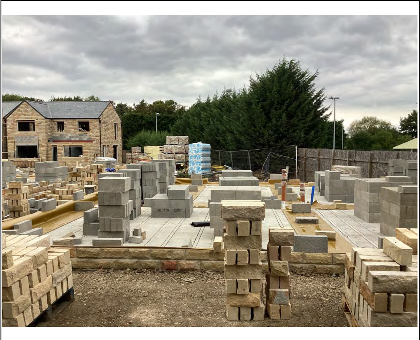
Overview of verified area - perimeter/internal walls
