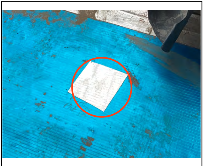
Remediated puncture within plot 37
