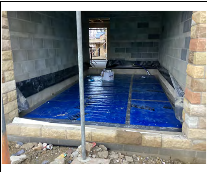
View showing completed Visqueen
