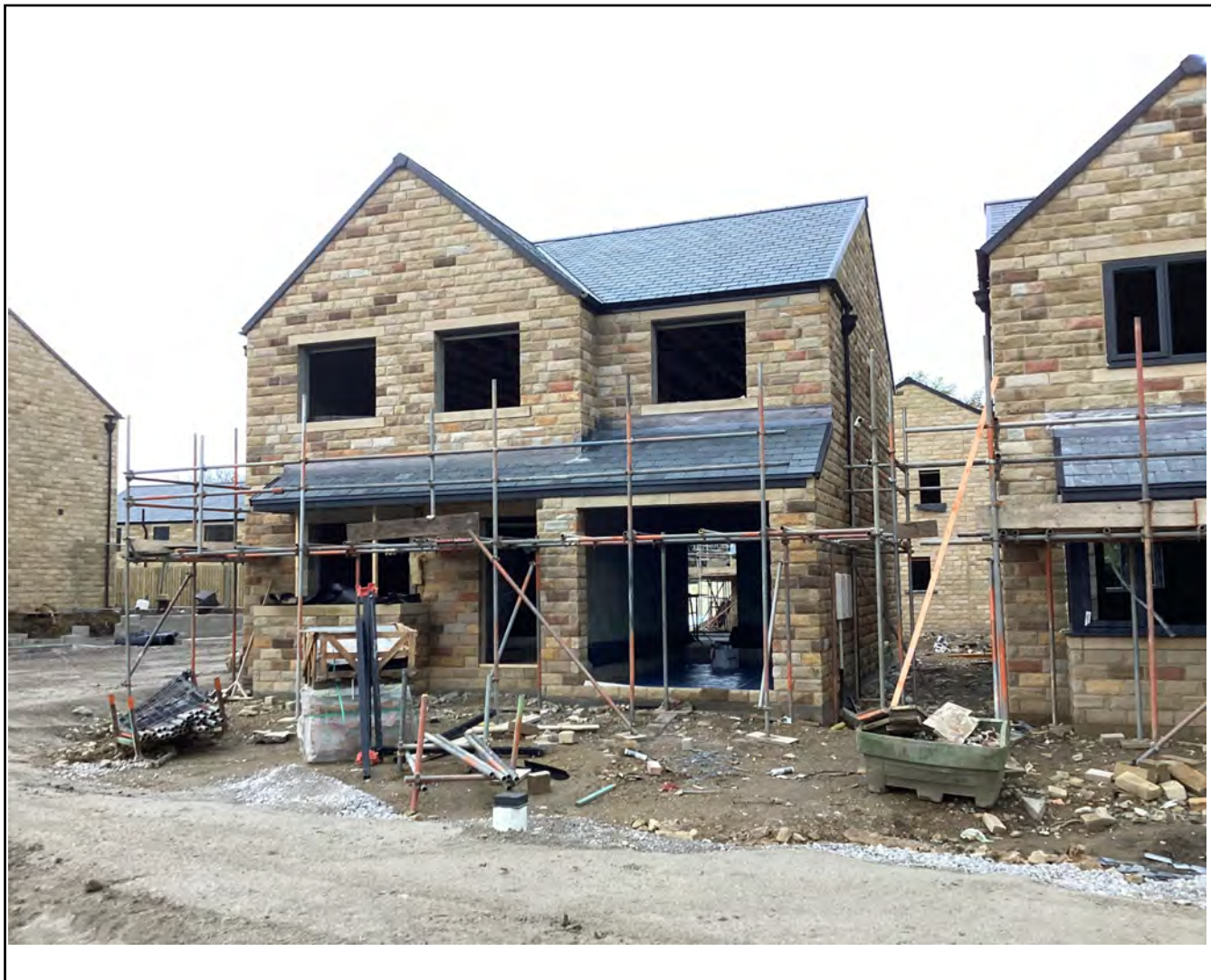
Overview of verified area - garage infill
