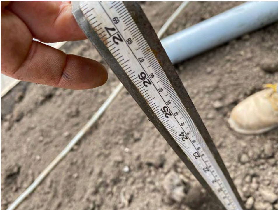
Close up of measuring bar used to prove 600mm depth.
