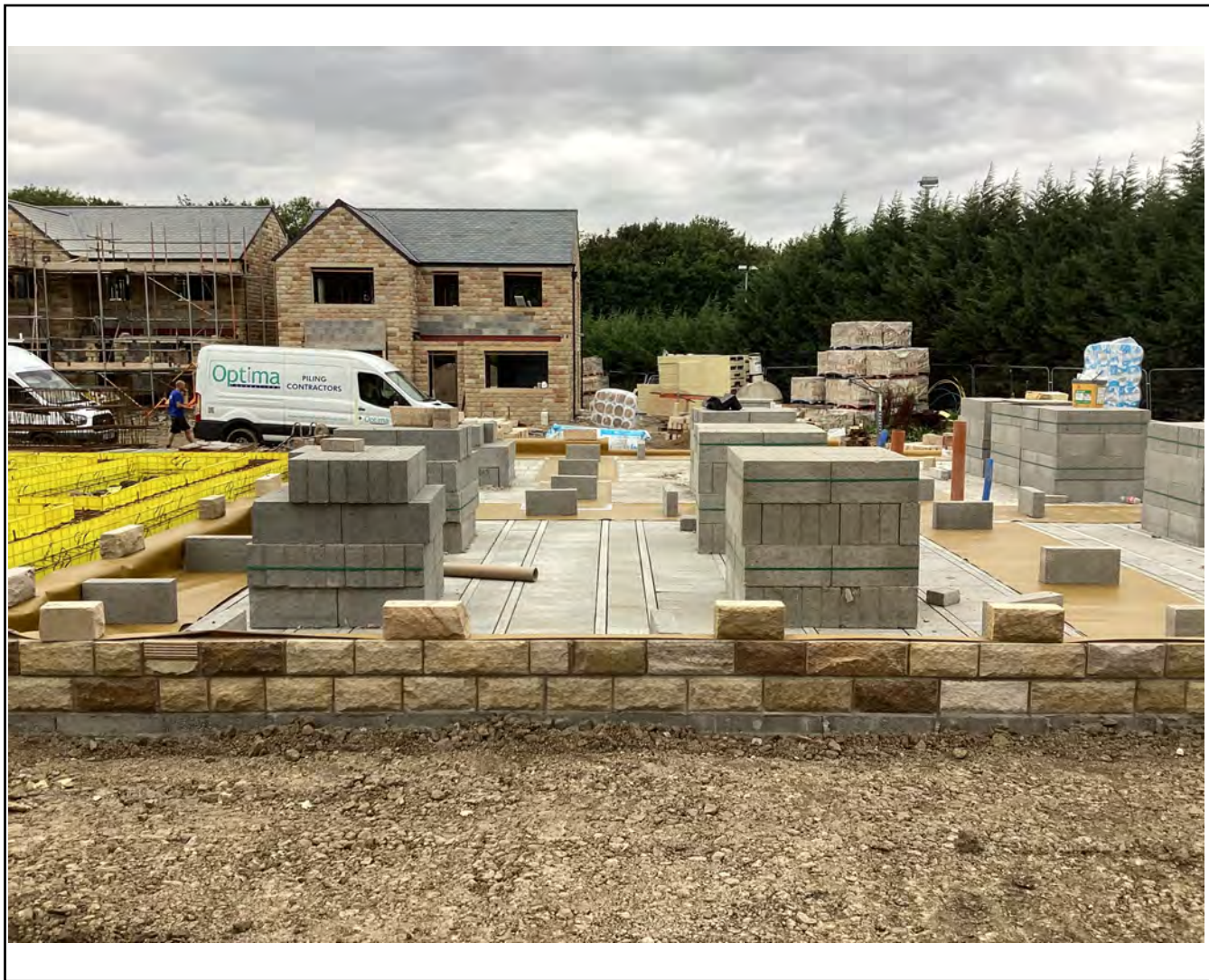
Overview of verified area - perimeter/internal walls
