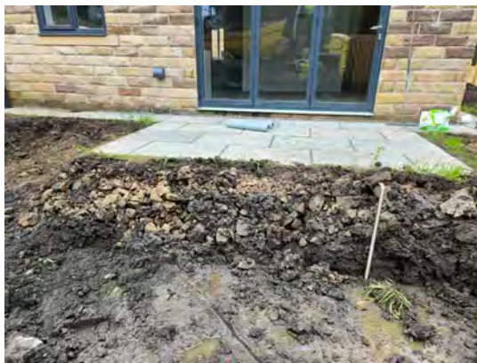
Plot 32 Removal of contaminated soil and Proving depth(L)
