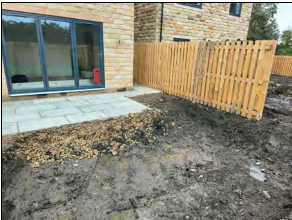
Plot 33 Removal of contaminated topsoil and depth proving(R)
