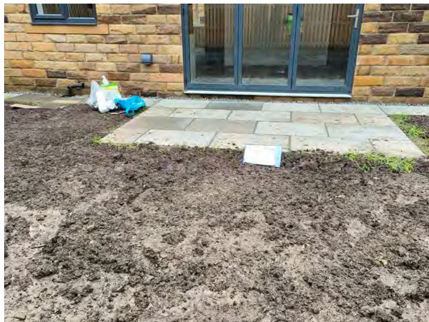
Plot 32 Refilled with new clean stockpile and sampled
