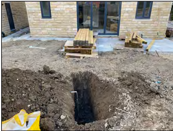
Rear Garden of Plot No 31 showing topsoil proving 600mm depth
