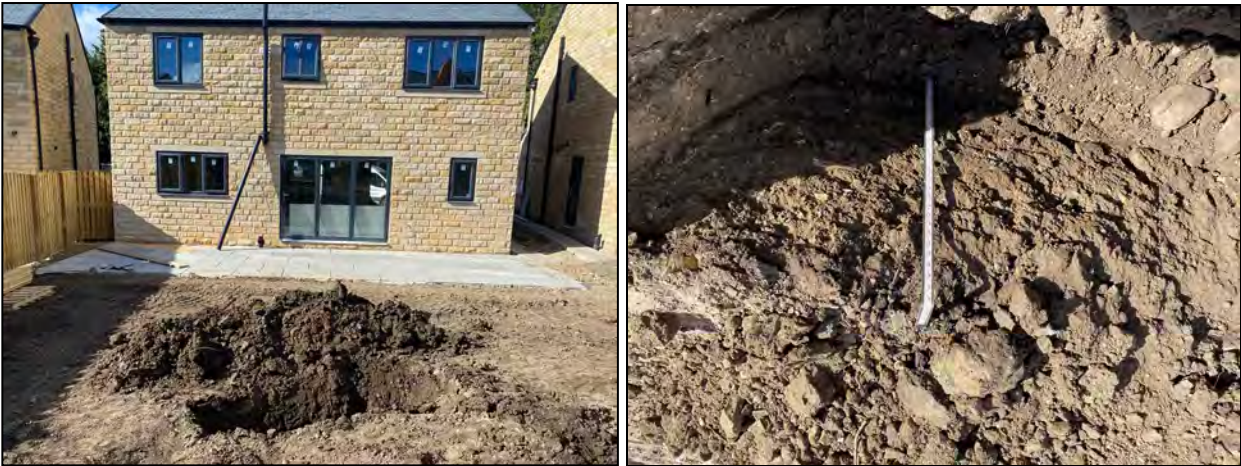
Rear Garden of Plot No 28 showing topsoil proving 600mm depth
