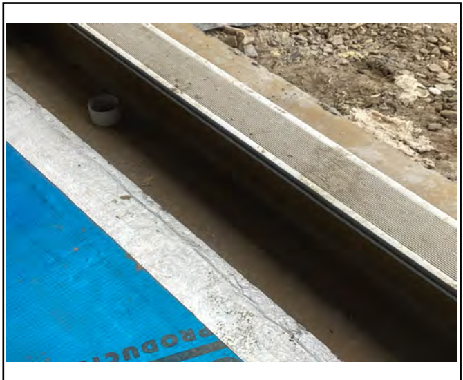
View showing the perimeter lap joint
