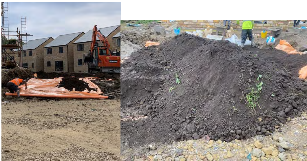
Figure 6 Topsoil stockpiles Hade Edge (left) and Shepley (right)
