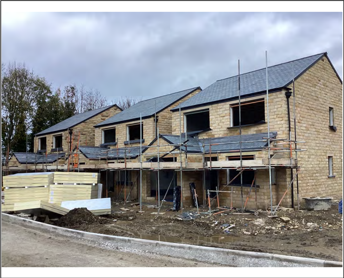
Overview of verified area
