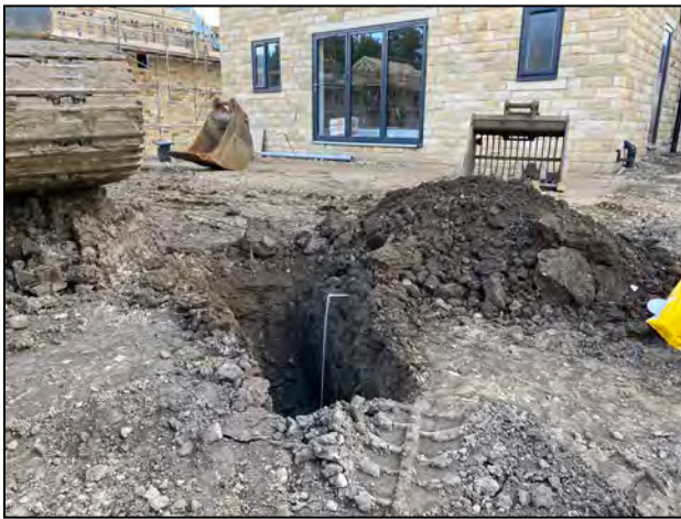
House Plot 30 rear view & Trial Pit proving 600mm of topsoil
