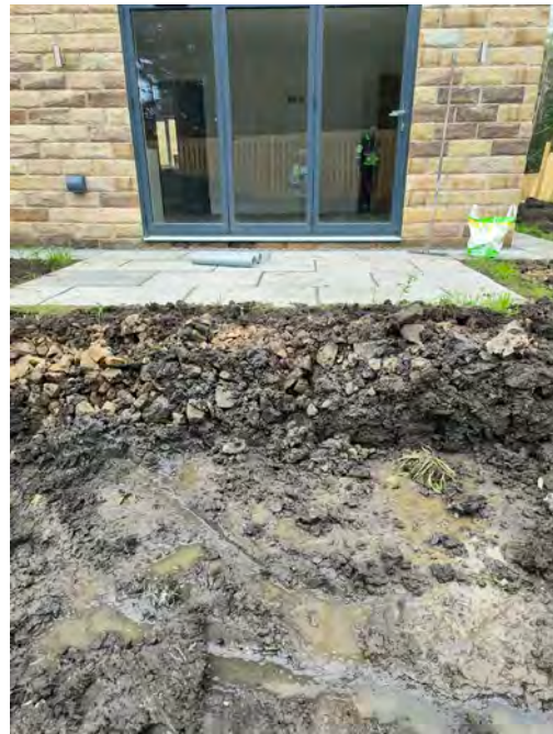
Plot 32 Removal of contaminated soil and Proving depth(L)
