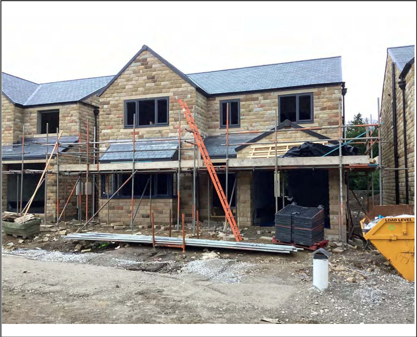
Overview of verified area - garage infill
