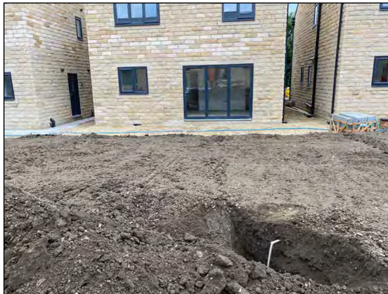
Associated Photo proving depth with 600mm tool used throughout
