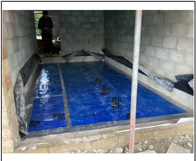
View showing completed Visqueen
