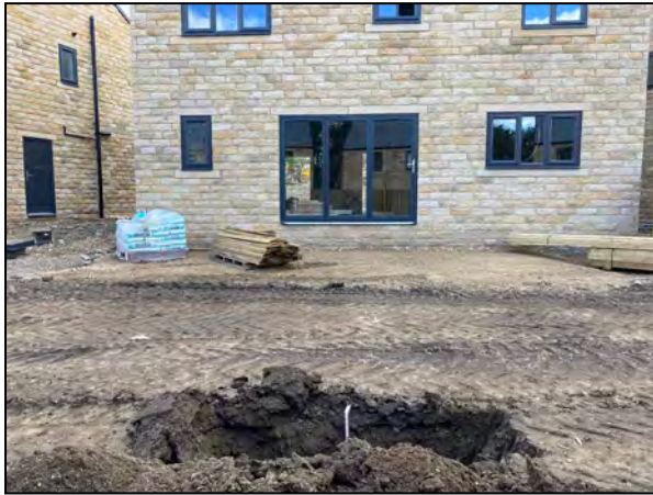
House Plot 29 rear view & Trial Pit proving 600mm of topsoil
