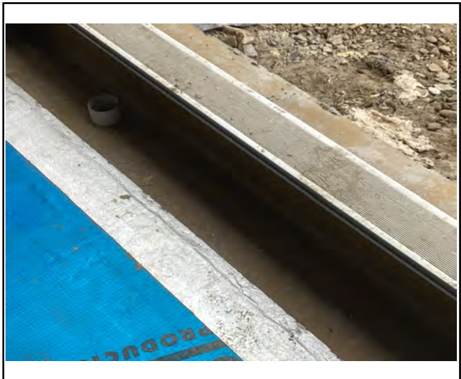
View showing the perimeter lap joint
