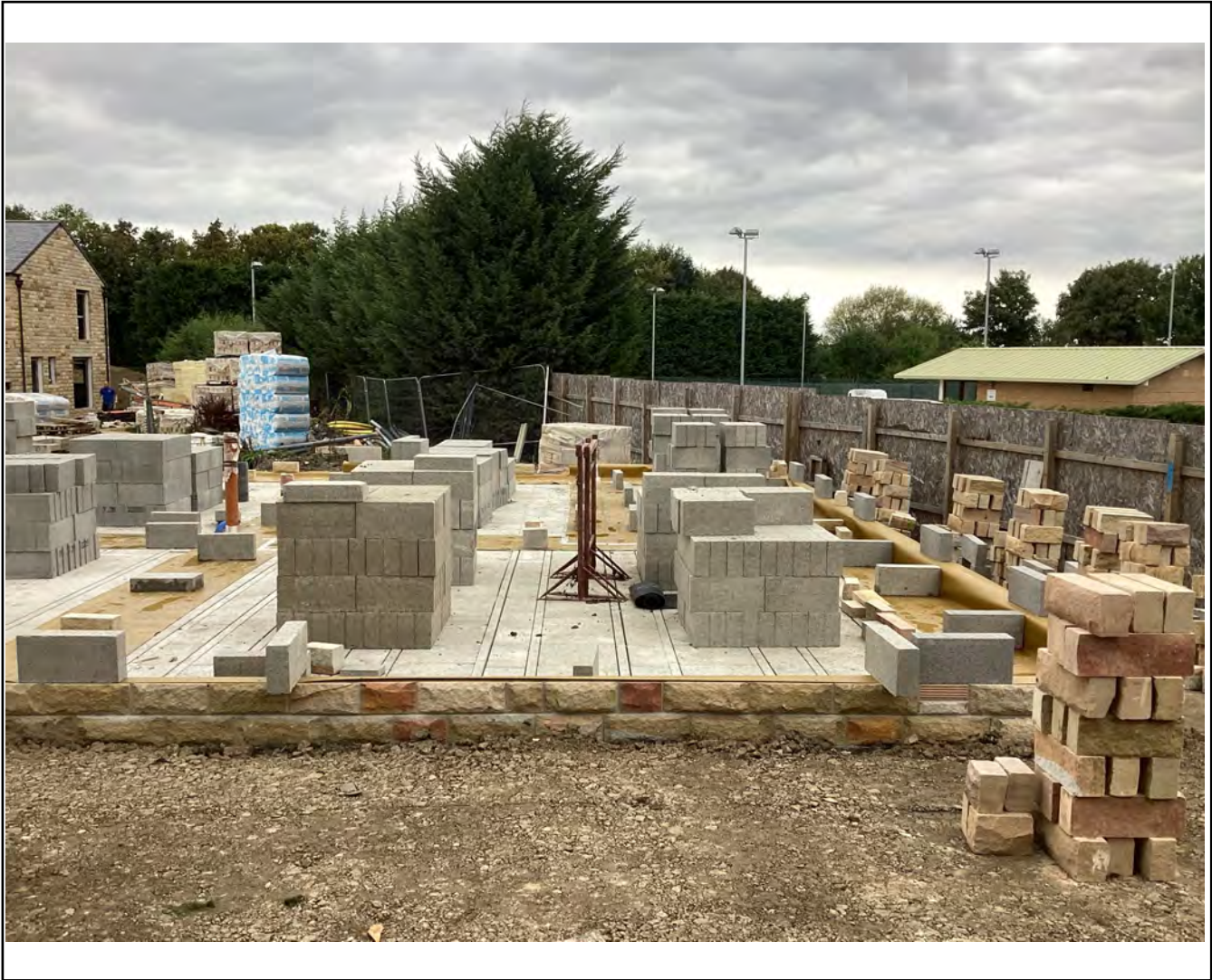
Overview of verified area - perimeter/internal walls
