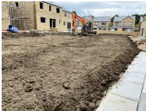
View over rear gardens of No 22-25 showing newly laid topsoil
