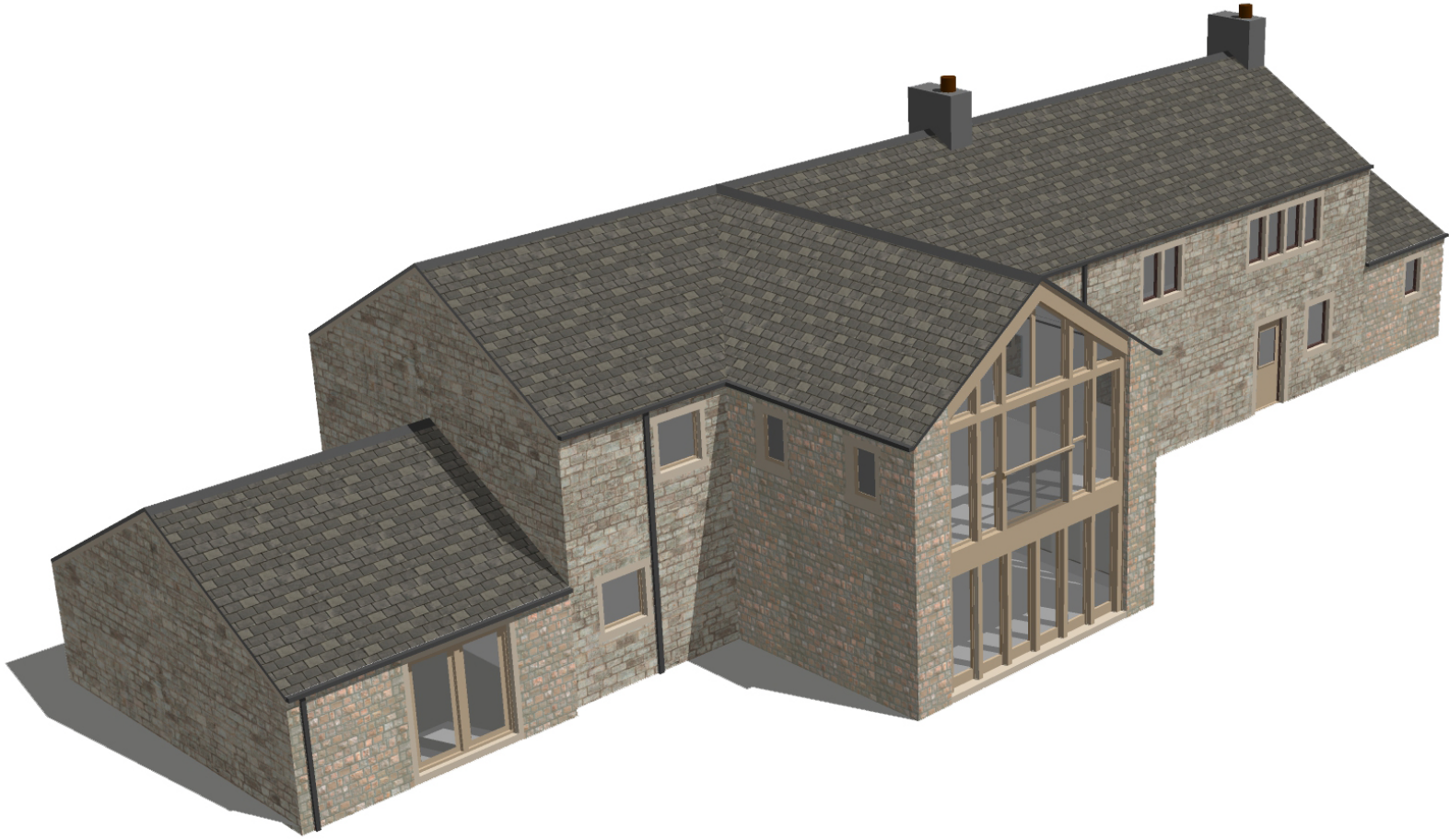
NORTH WEST VIEW
