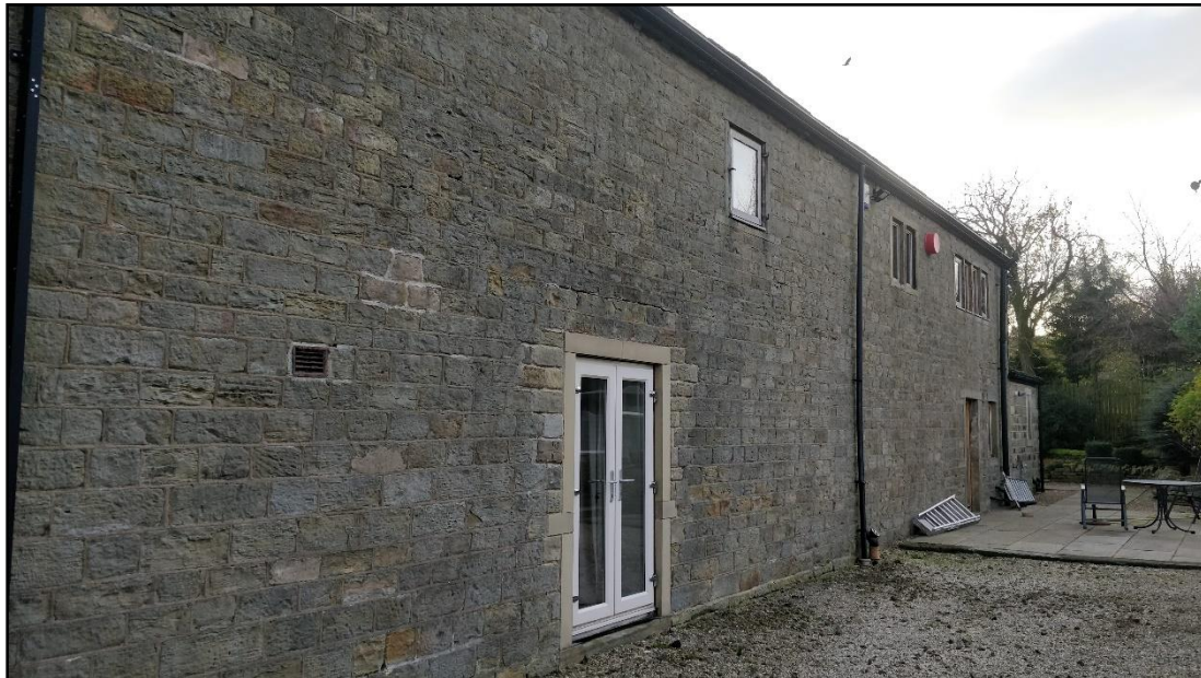
Photograph showing the existing rear/west elevation
