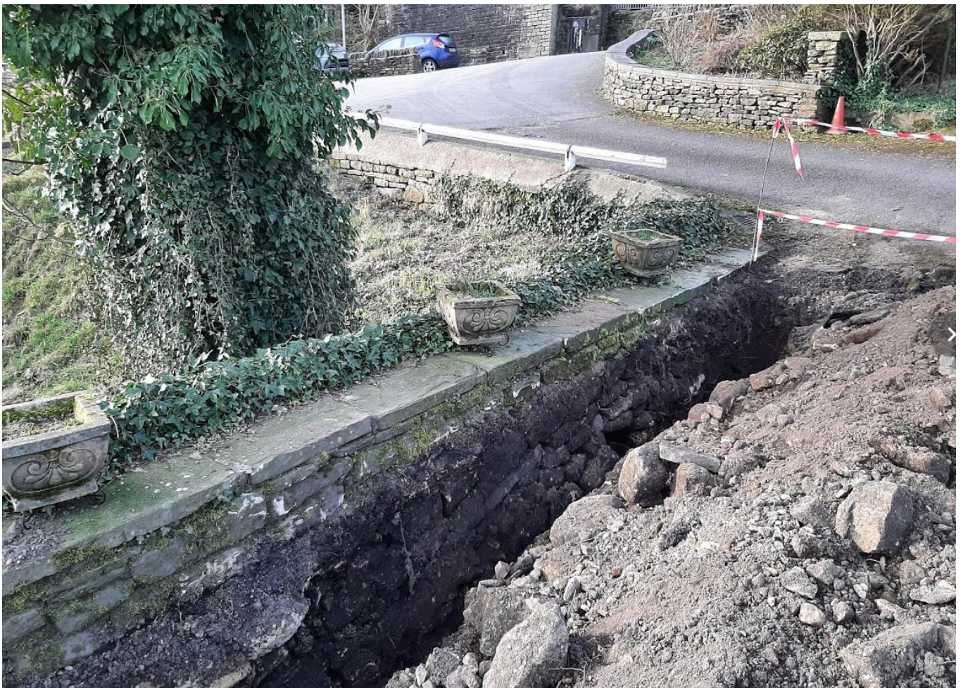
Inspection trench from north
