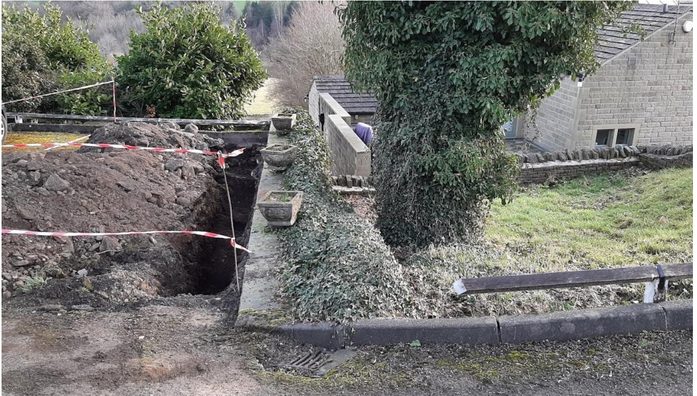
Inspection trench from south west
