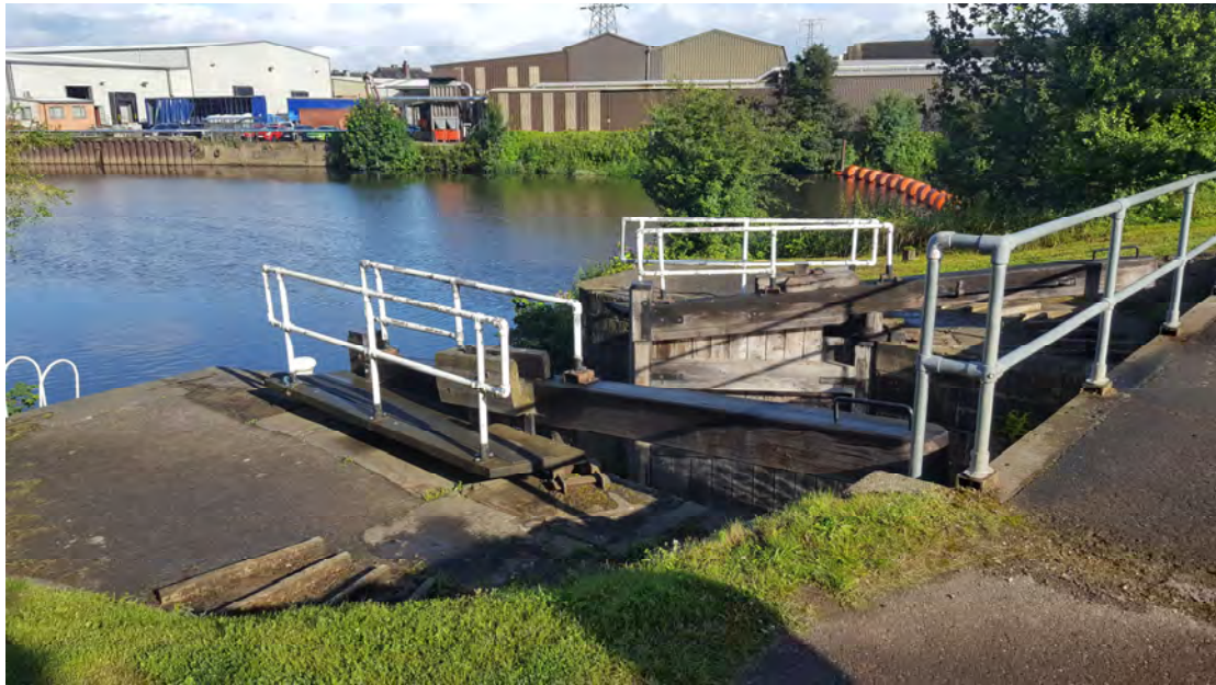
Thornhill Lock & Barrier (upstream of site)
