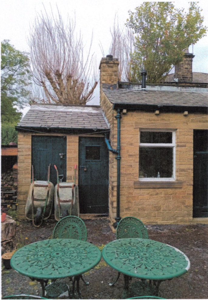
ADDED SINGLE STOREY EXTENSION
