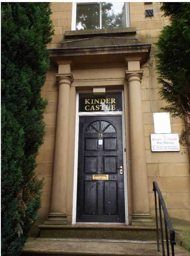
The main entrance to the north elevation
