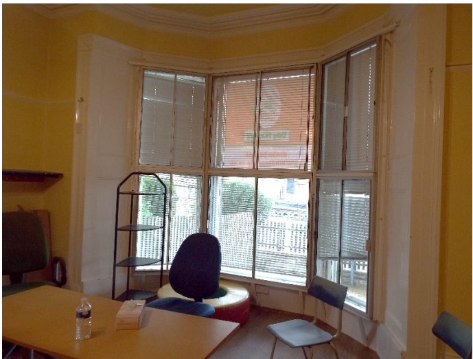
Canted bay to classroom 2
