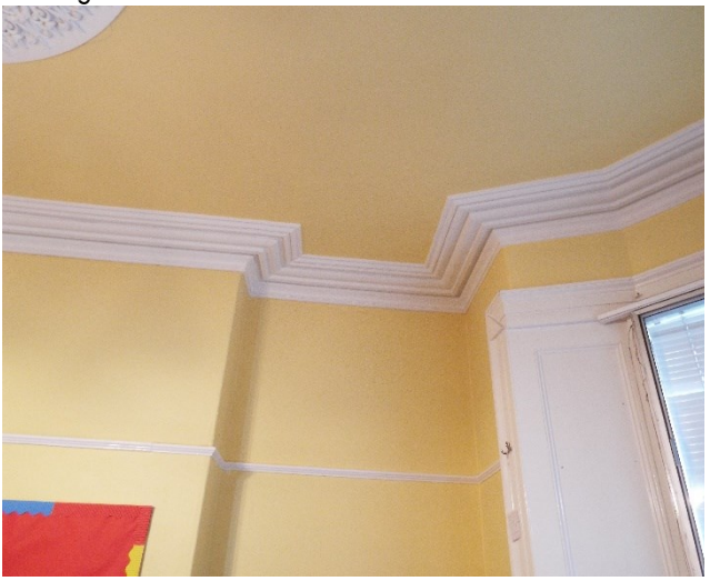
Plaster cornice classroom 2
