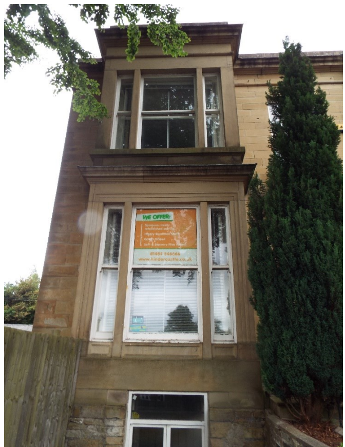
Windows to the east side of the north elevation
