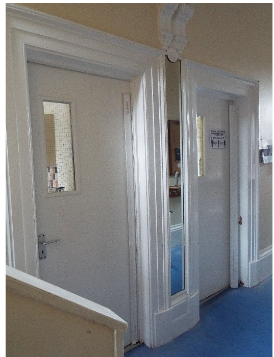
Timber door surround to the hallway
