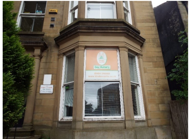
Canted bay to the ground floor
