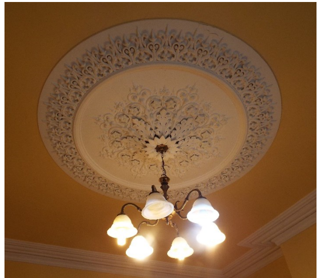
Ceiling rose to classroom 2
