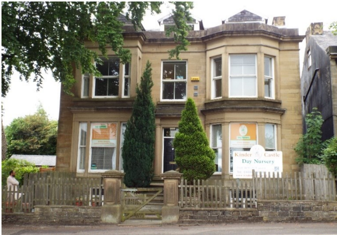
The northeast elevation
