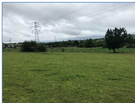
Image 18. P.O.C site (looking across S field compartment)
