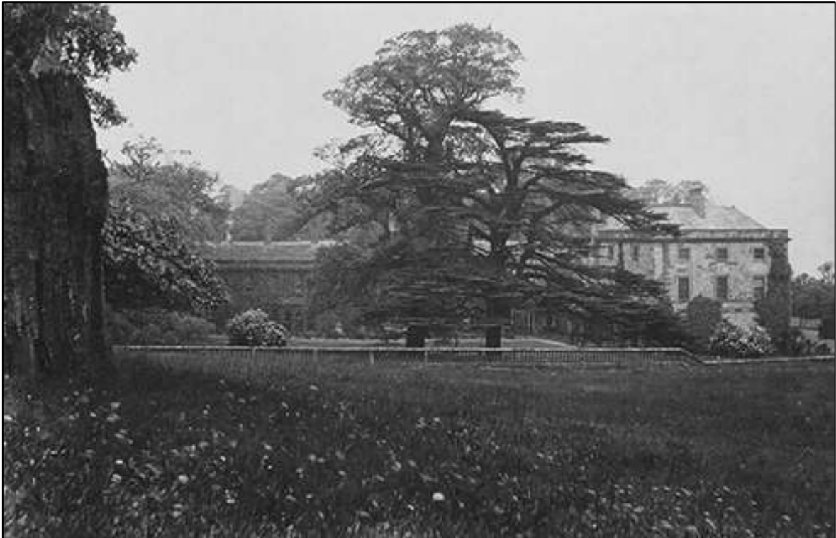
FIGURE 4: VIEW OF THE HOUSE FROM THE SOUTH (FROM WWW.LOSTHERITAGE.ORG.UK ).
