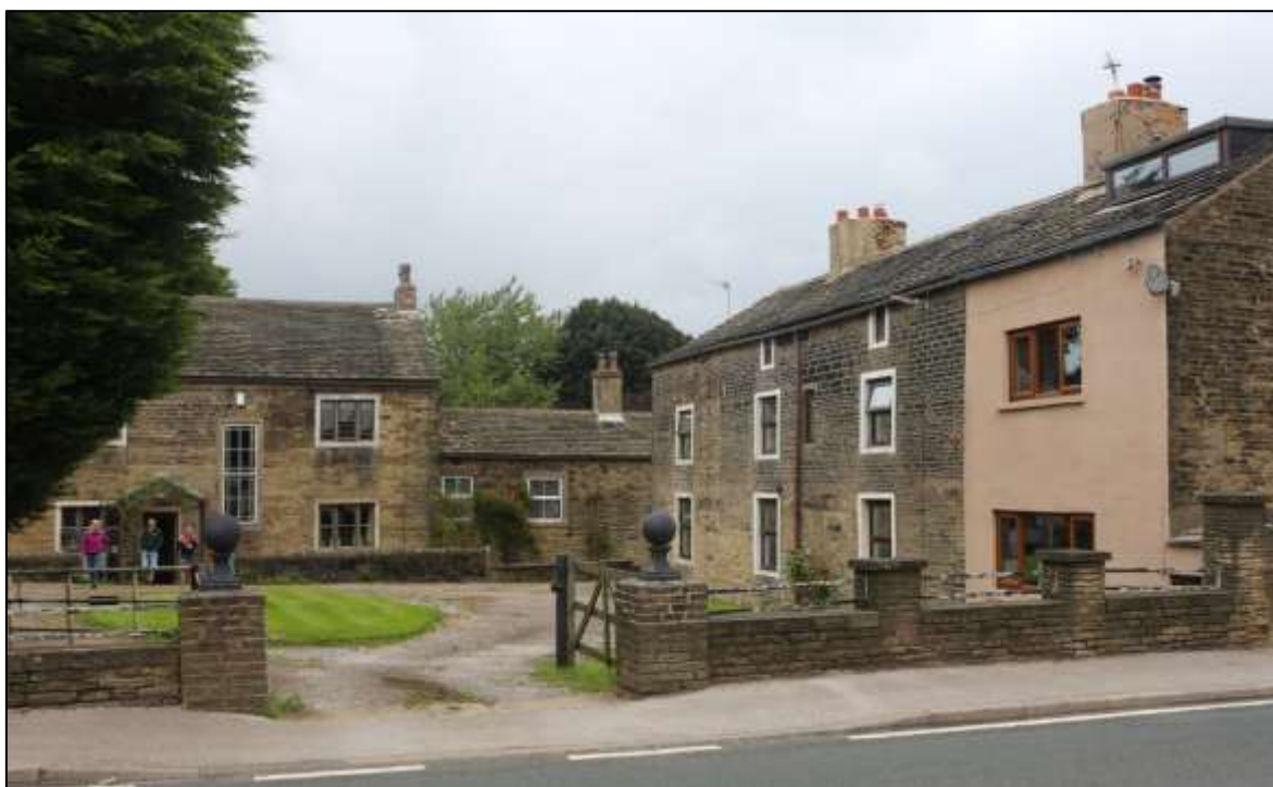
FIGURE 44: ROOKERY FARM; VIEWED FROM THE A642 TO THE SOUTH.
