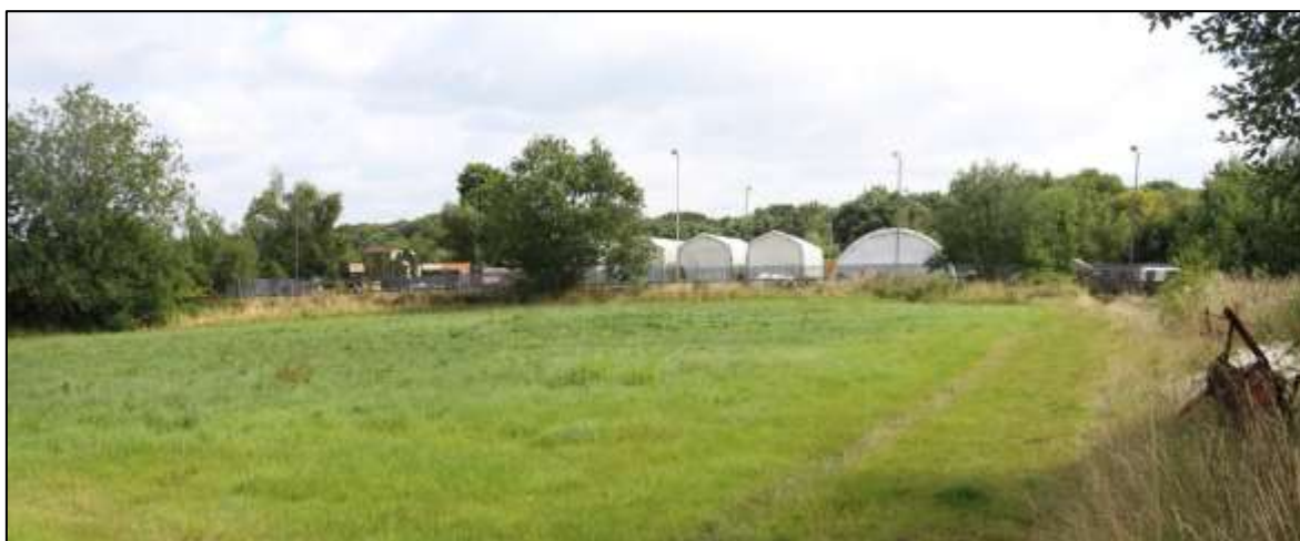
FIGURE 49: THE WESTERN EDGE OF THE CONSERVATION AREA WITH FIELD P IN THE FOREGROUND; VIEWED FROM THE WEST.
