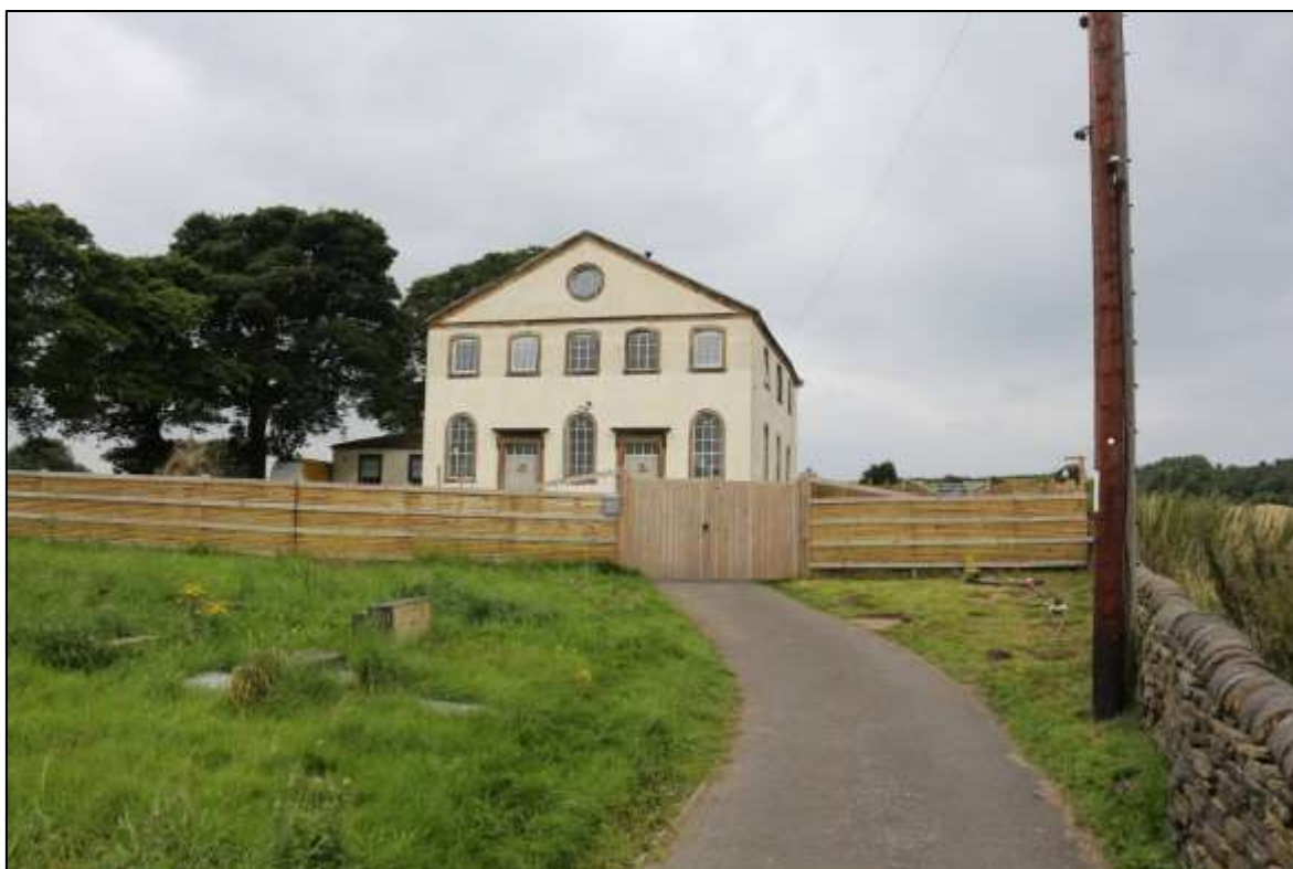
FIGURE 45: THE SOUTH FRONT OF THE CHAPEL; VIEWED FROM THE SOUTH.
