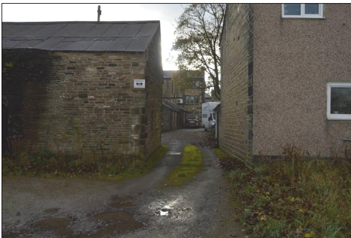
Photograph 11: Stone quoined corners and east gable features (facing north west).
