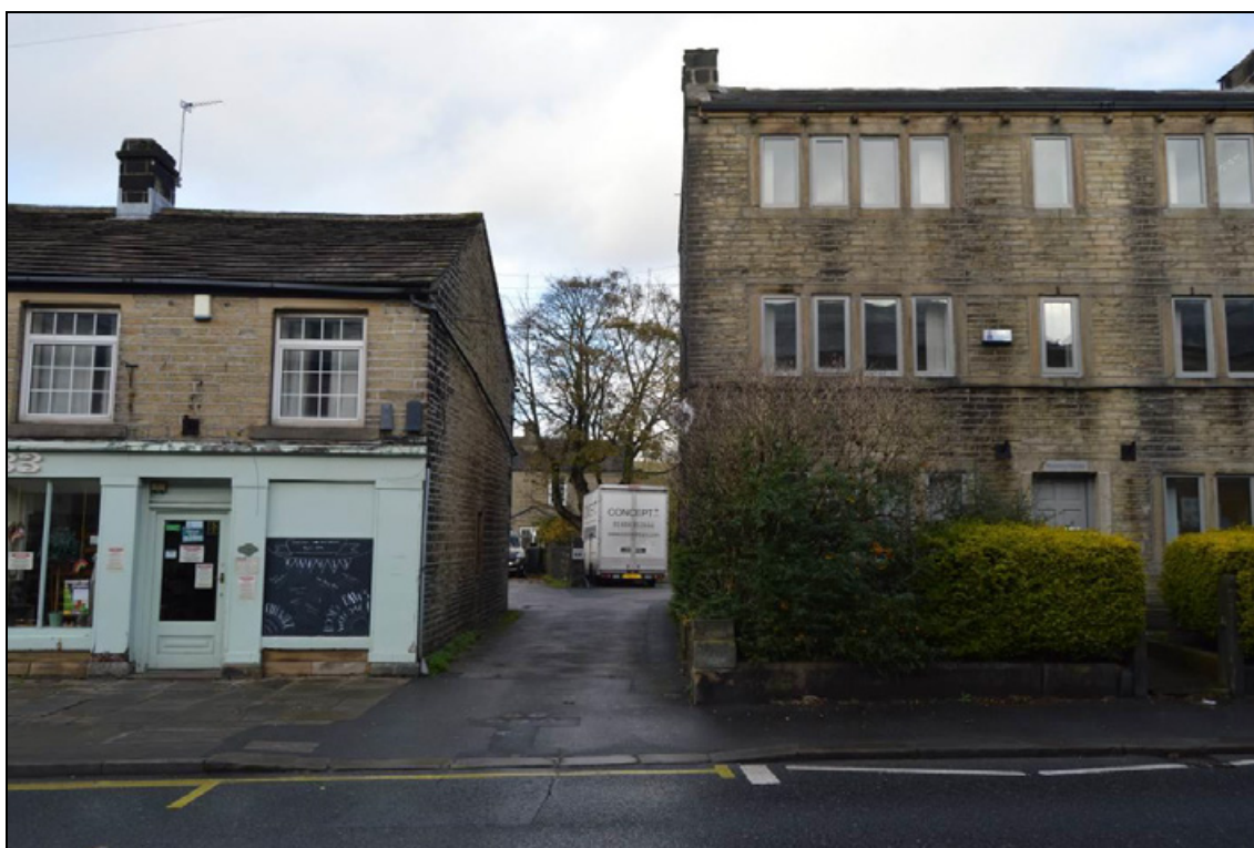
Photograph 3: View from Huddersfield Road (looking north) through to the rear extent of the site.
