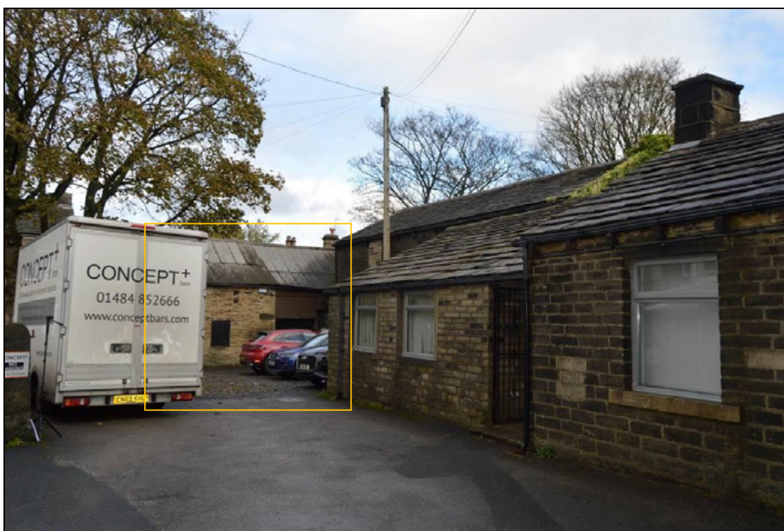
Photograph 4: The rear yard area of Midway House (looking north east), the barn (Building 1) indicated.
