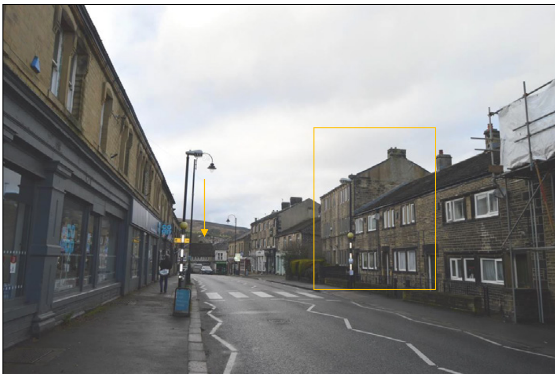
Photograph 1: Huddersfield Road approaching from the east towards the Market Place (looking north west, with Wessenden Head in the background: yellow arrow) with the Midway House (Building 1), indicated.
