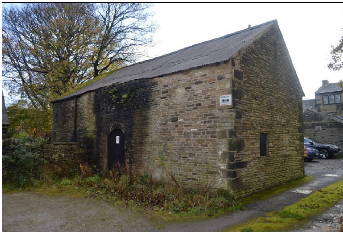
Photograph 10: North aspects of the barn (facing south east). Scale 0.5m.
