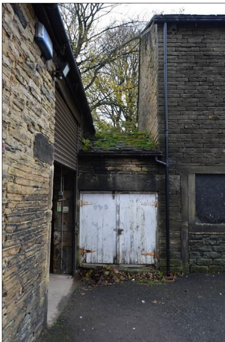
Photograph 23: Building 2 from the rear yard.
