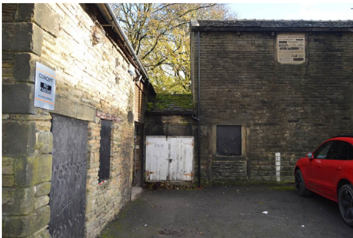
Photograph 24: Building 2 adjoining the two barns (facing east).
