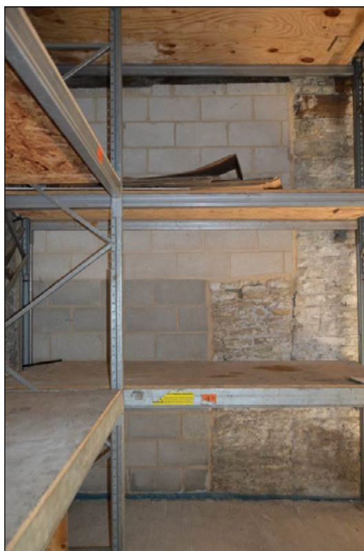
Photograph 20: Blocked internal doorway in north elevation to demolished north extension.
