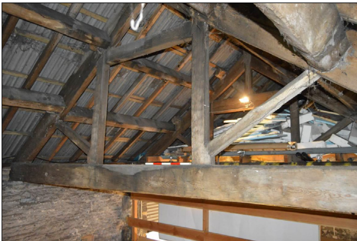
Photograph 21: Queen-post roof trusses to roof of barn. Scale 0.5m.
