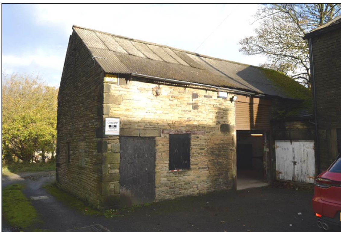
Photograph 9: South aspect of the barn (facing north). Scale 0.5m.
