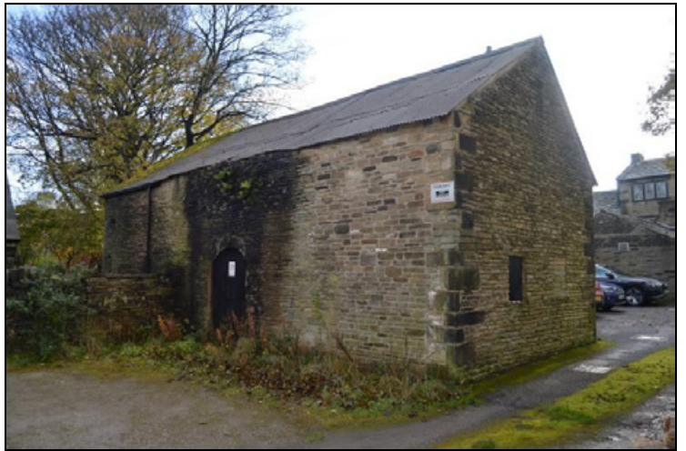
View of the barn to the rear of Midway House, Meltham
