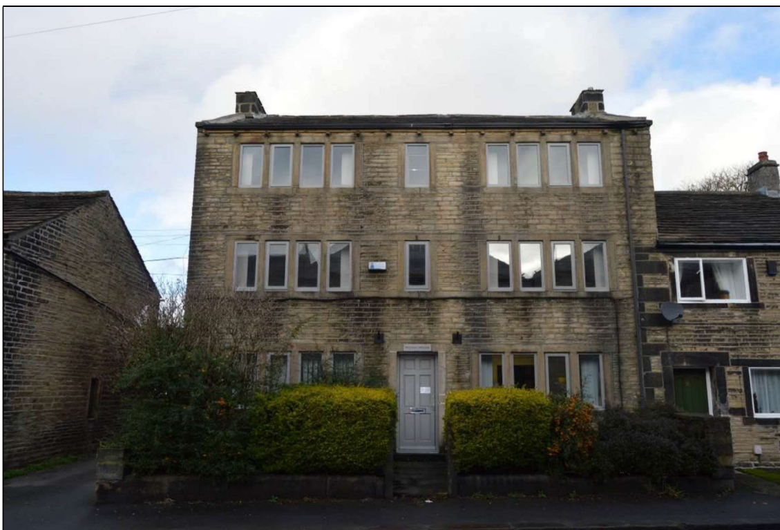
Photograph 8: Front aspect of Midway House from Huddersfield Road (facing north).
