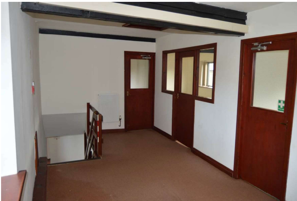
Photograph 29: Second floor landing. Scale 0.5m.
