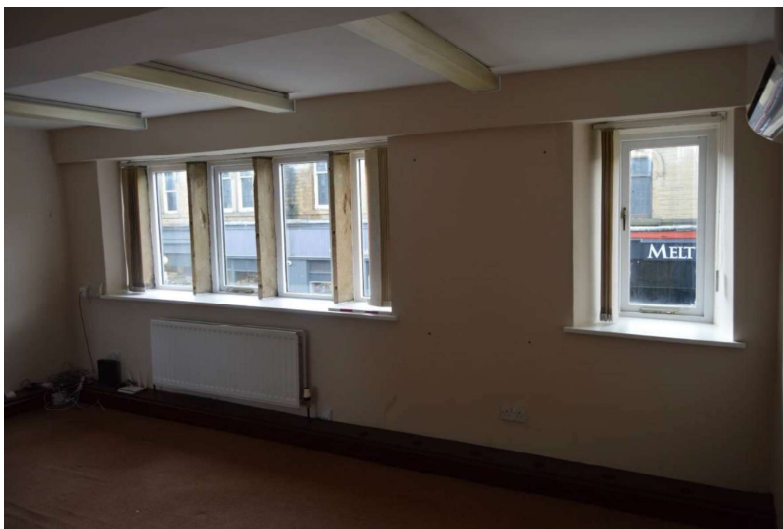
Photograph 28: First floor room front aspect. Scale 0.5m.
