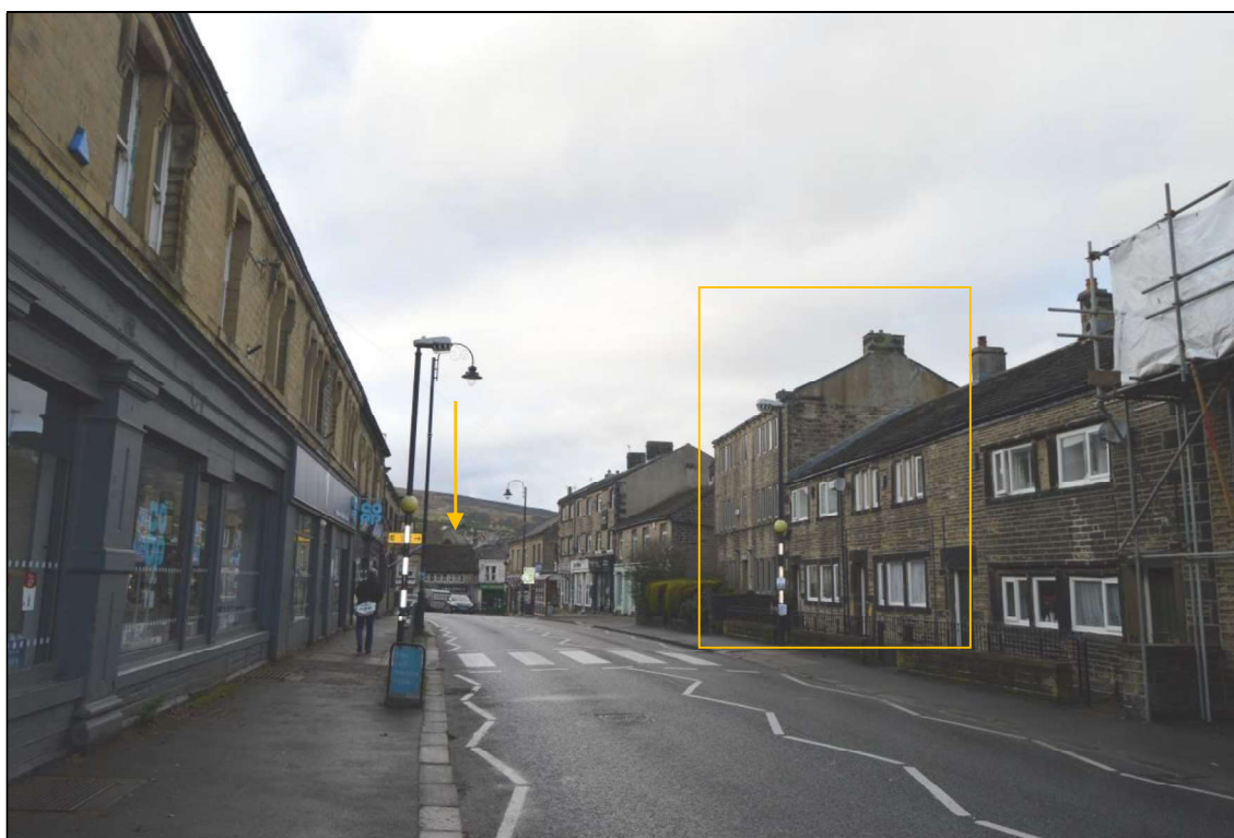
Photograph 1: Huddersfield Road approaching from the east towards the Market Place (looking north west, with Wessenden Head in the background) with the Midway House (Building 1, also indicated).
