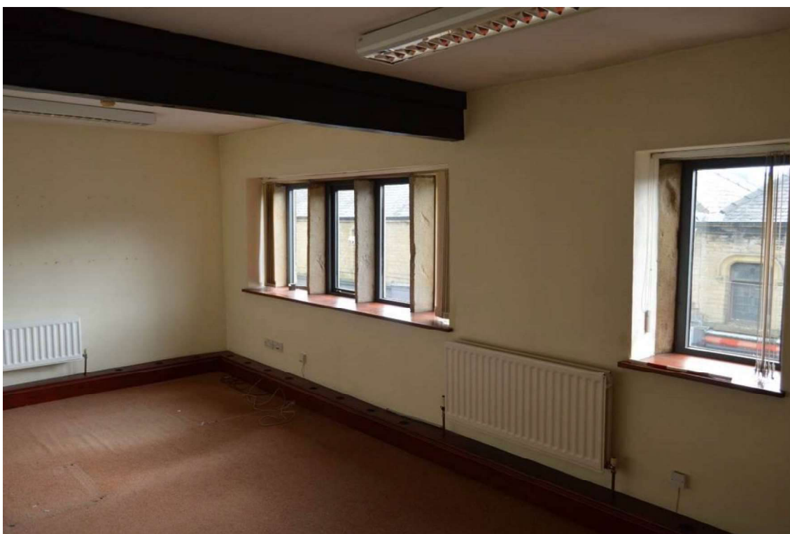
Photograph 30: Second floor room with windows to front aspect. Scale 0.5m.
