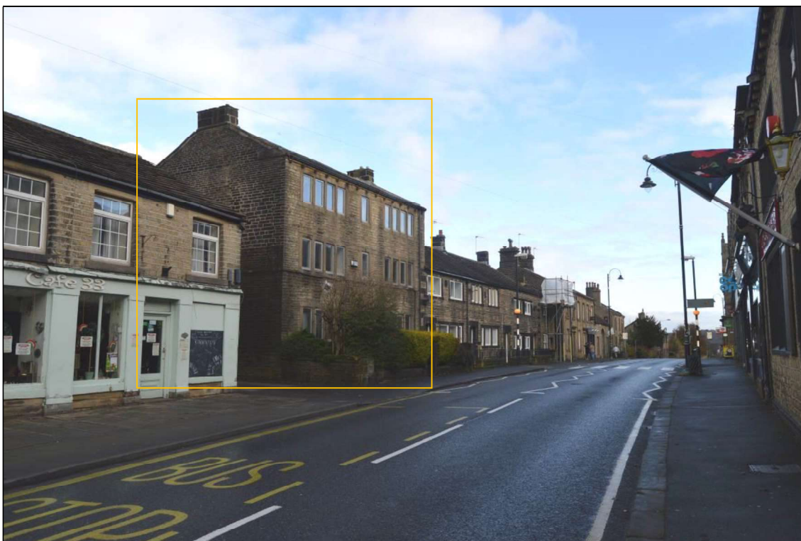
Photograph 2: Huddersfield Road approaching along from the west (looking north east) east towards the Market Place (looking north west) with the Midway House (building 1, indicated).
