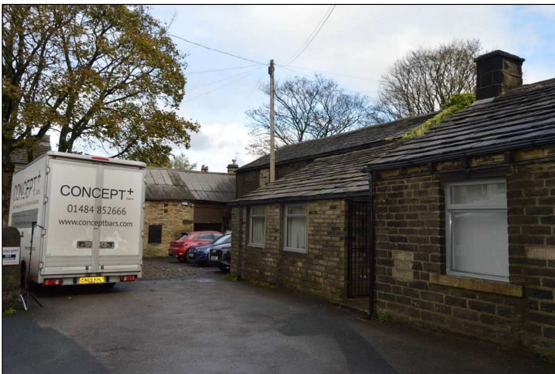
Photograph 4: The rear yard area of Midway House (looking north east).
