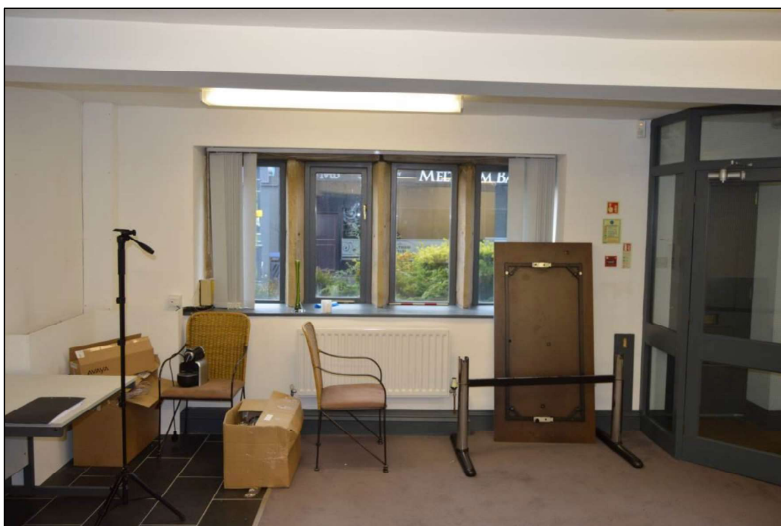
Photograph 22: Mullioned windows to the front of the building, from the east, ground floor room. Scale 0.5m.
