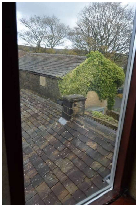
Photograph 32: Capped chimney stack of building 2.
