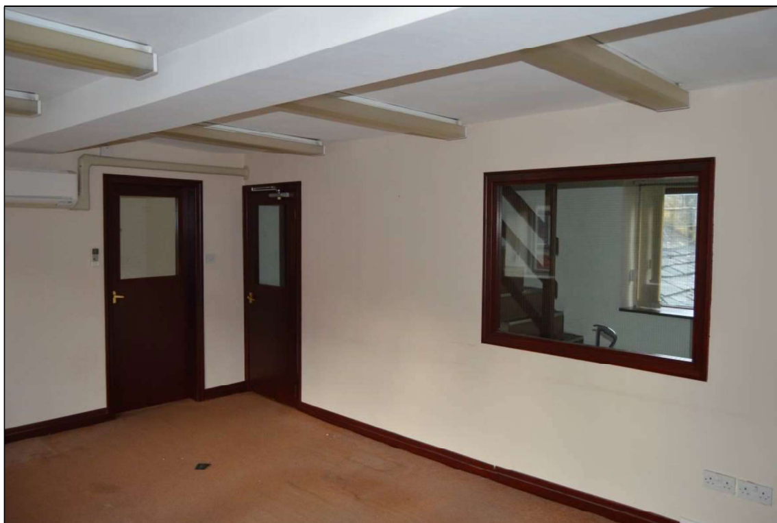
Photograph 27: First floor partitioned room. Scale 0.5m.
