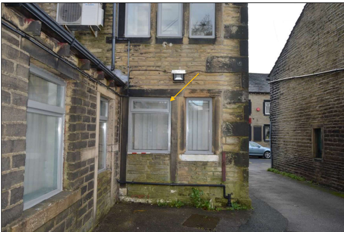
Photograph 15: View of rear elevation with former doorway (indicated).
