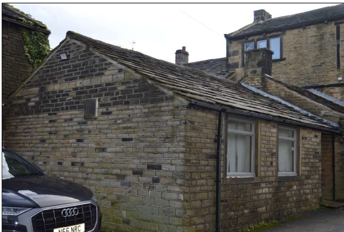
Photograph 35: Exterior to building 3.
