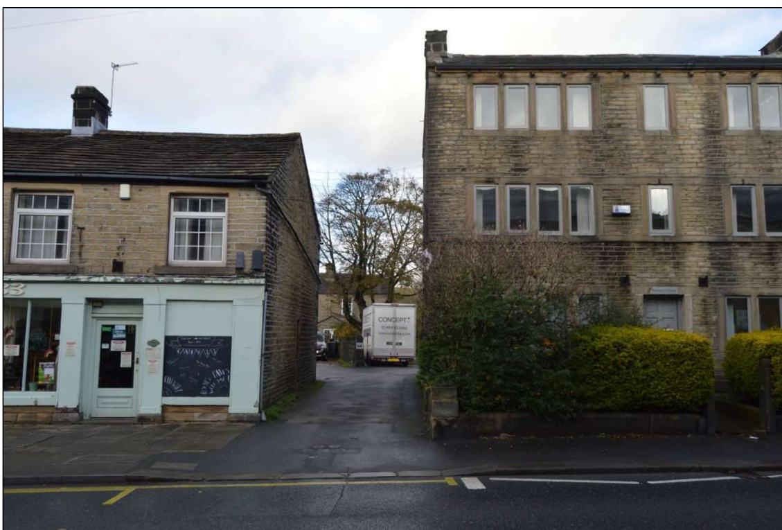
Photograph 3: View from Huddersfield Road (looking north) through to the rear extents of the site.
