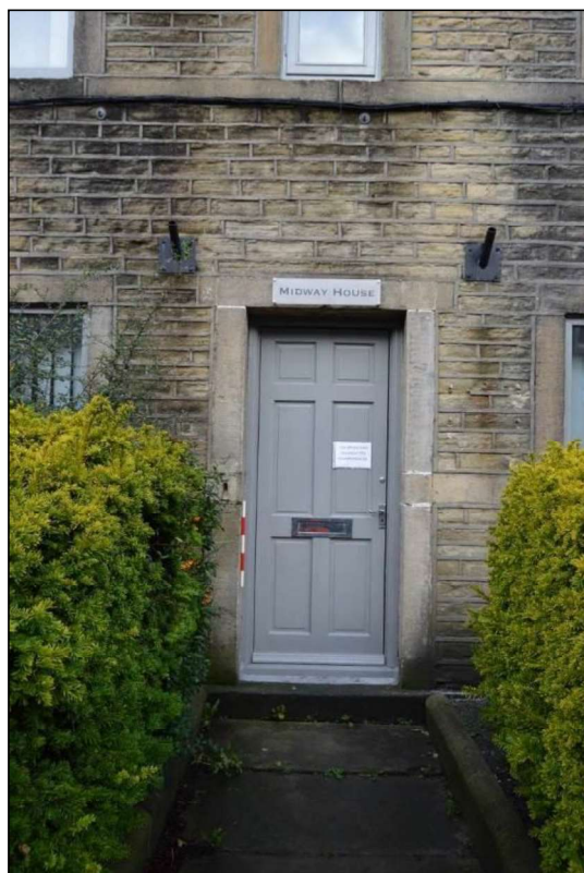
Photograph 10: Front door (facing north). Scale 0.5m.
