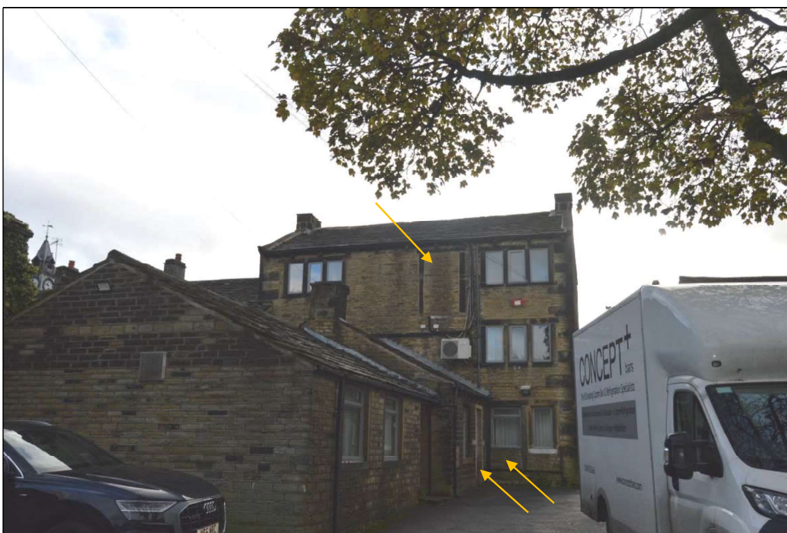
Photograph 13: Rear aspect of Midway house (facing south), with its series of extensions to foreground. Historic, blocked doorway apertures are indicated.
