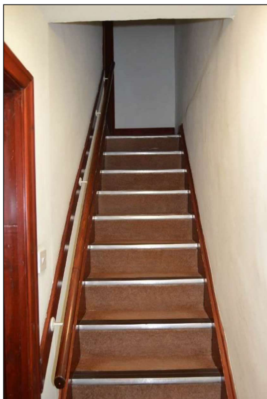
Photograph 25: Stairs from ground floor to first floor landing.
