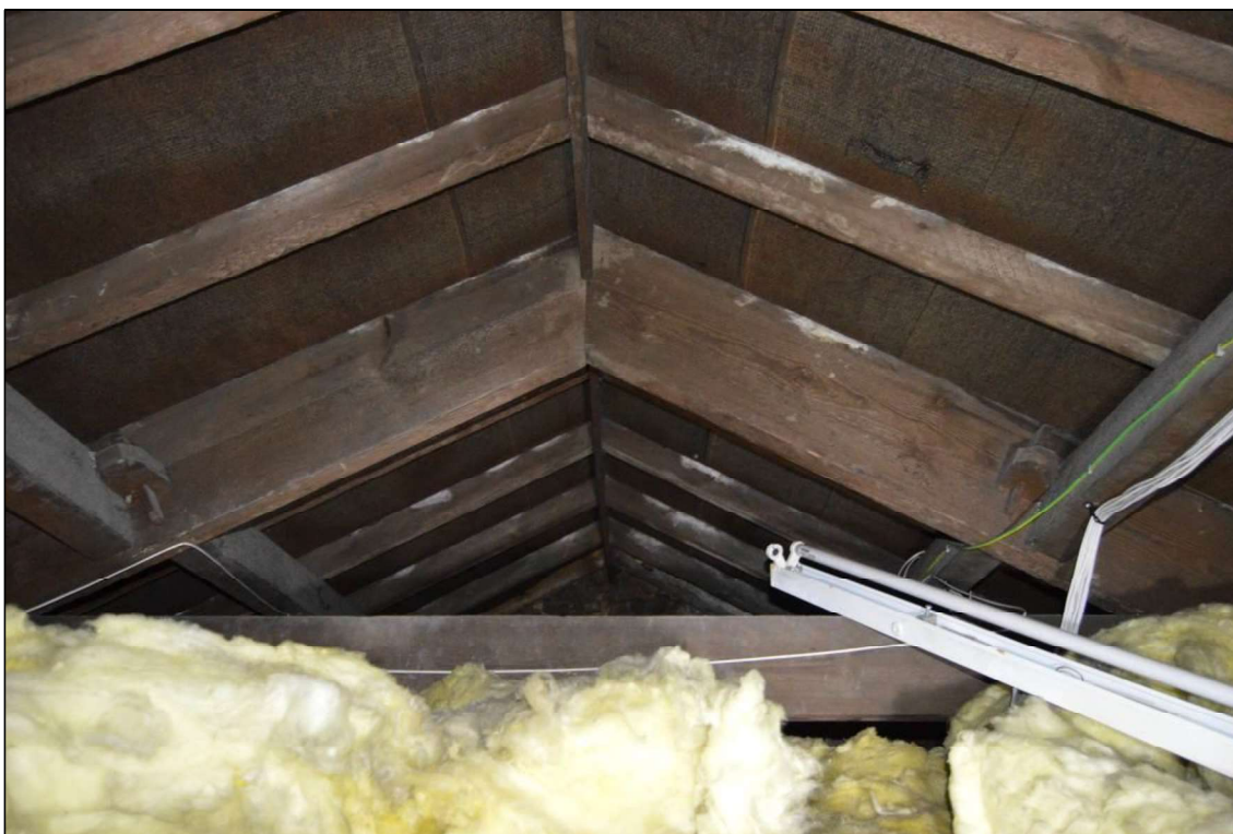
Photograph 34: Roof structure to Building 2.
