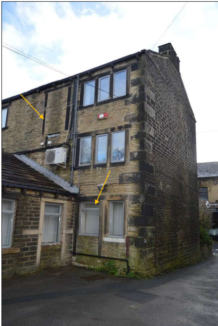
Photograph 14: North wall (facing south) with hoist door and possible cottage doorway (indicated) surrounds in situ .
