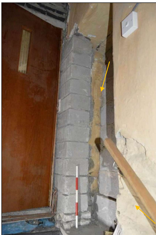
Photograph 20: Former external doorway (stone jamb in situ indicated) in the north elevation now internalised behind the later extension. Scale 0.5m.
