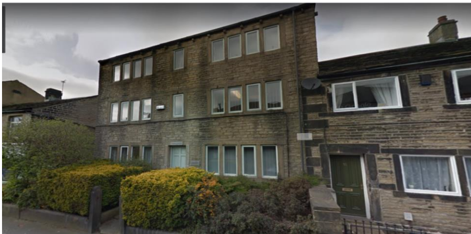
Photograph 1: Midway House from site frontage
