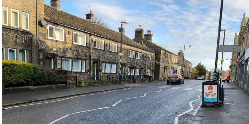
Photograph 4: Pedestrian crossing facilities in the vicinity of the site
