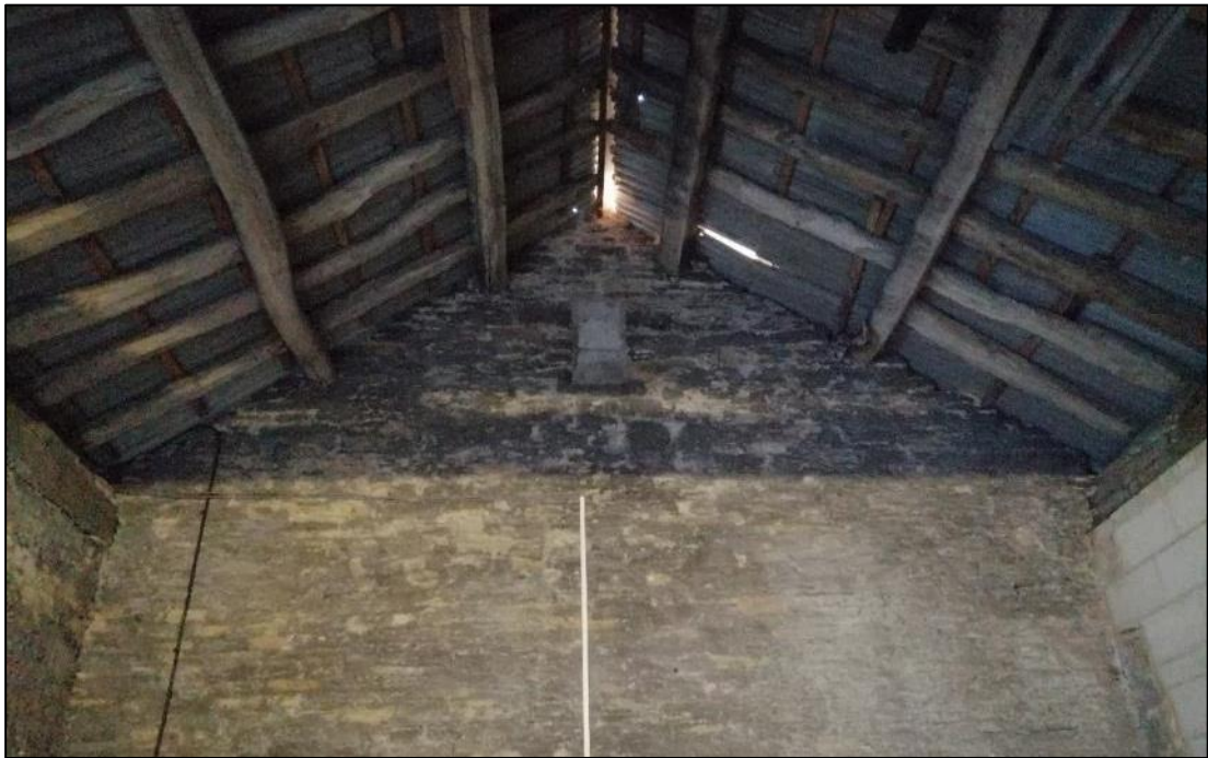
Plate 8. Inside of barn
