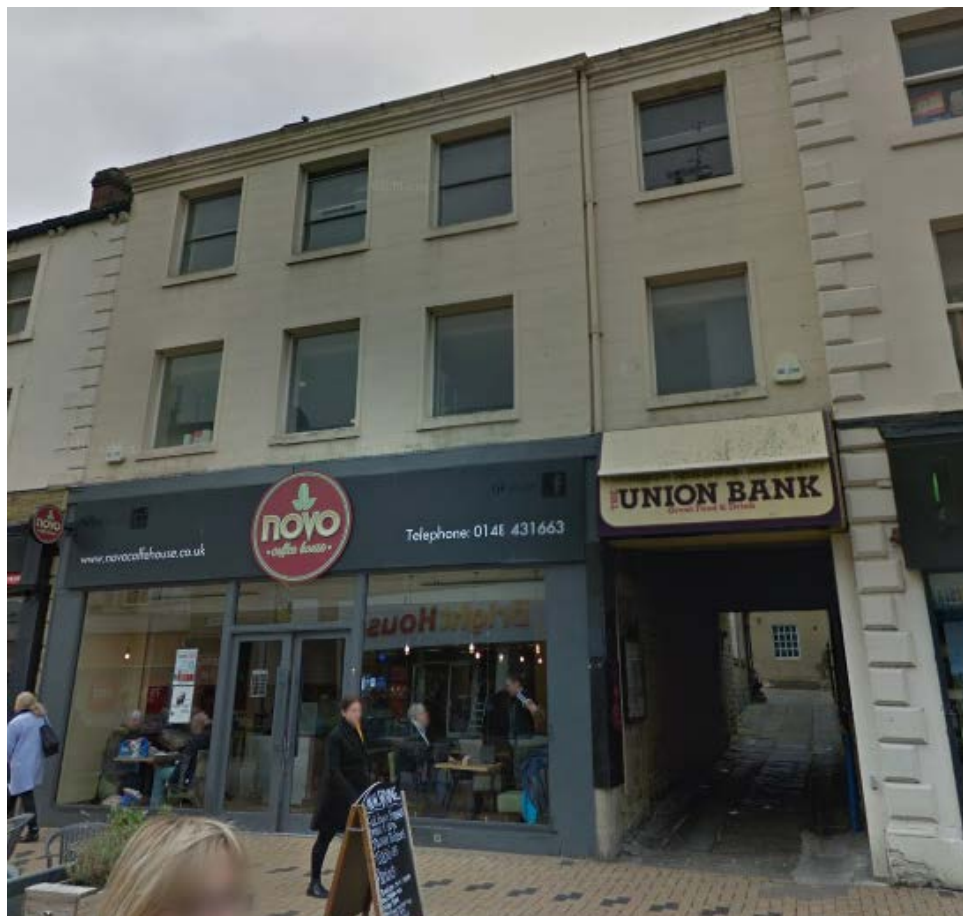
Photo showing the existing front facade of the property
