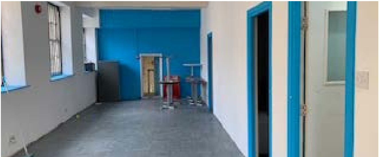
Photo showing the current conditions of the first floor
