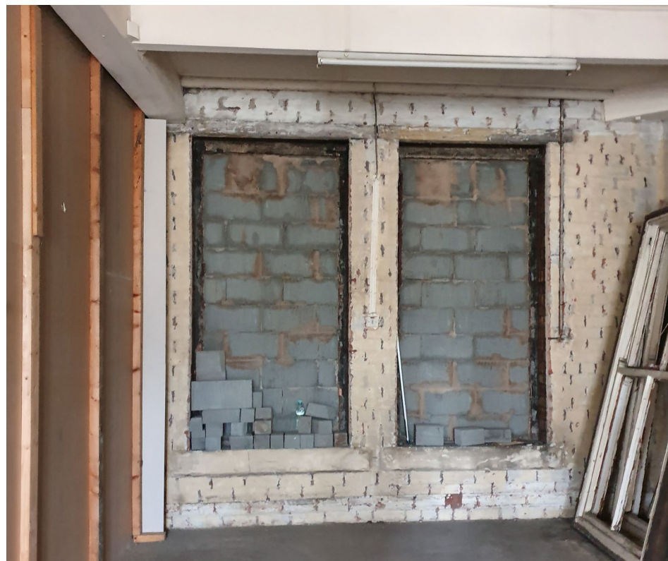
Figures 6.10.21 Site photographs of Corporation Street Level 2 (BDP 2021)
