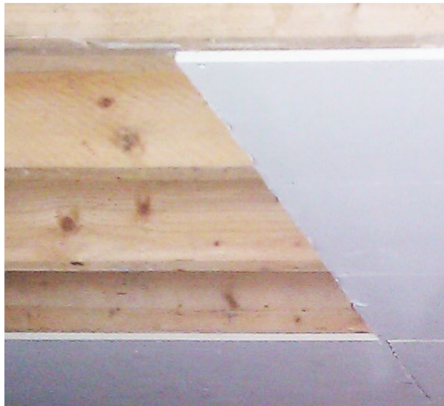
Ceiling finishes - Plasterboard
