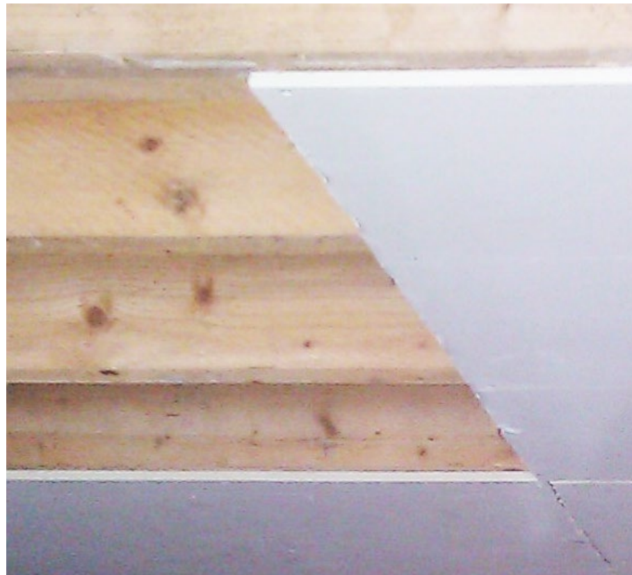
Ceiling finishes - Plasterboard
