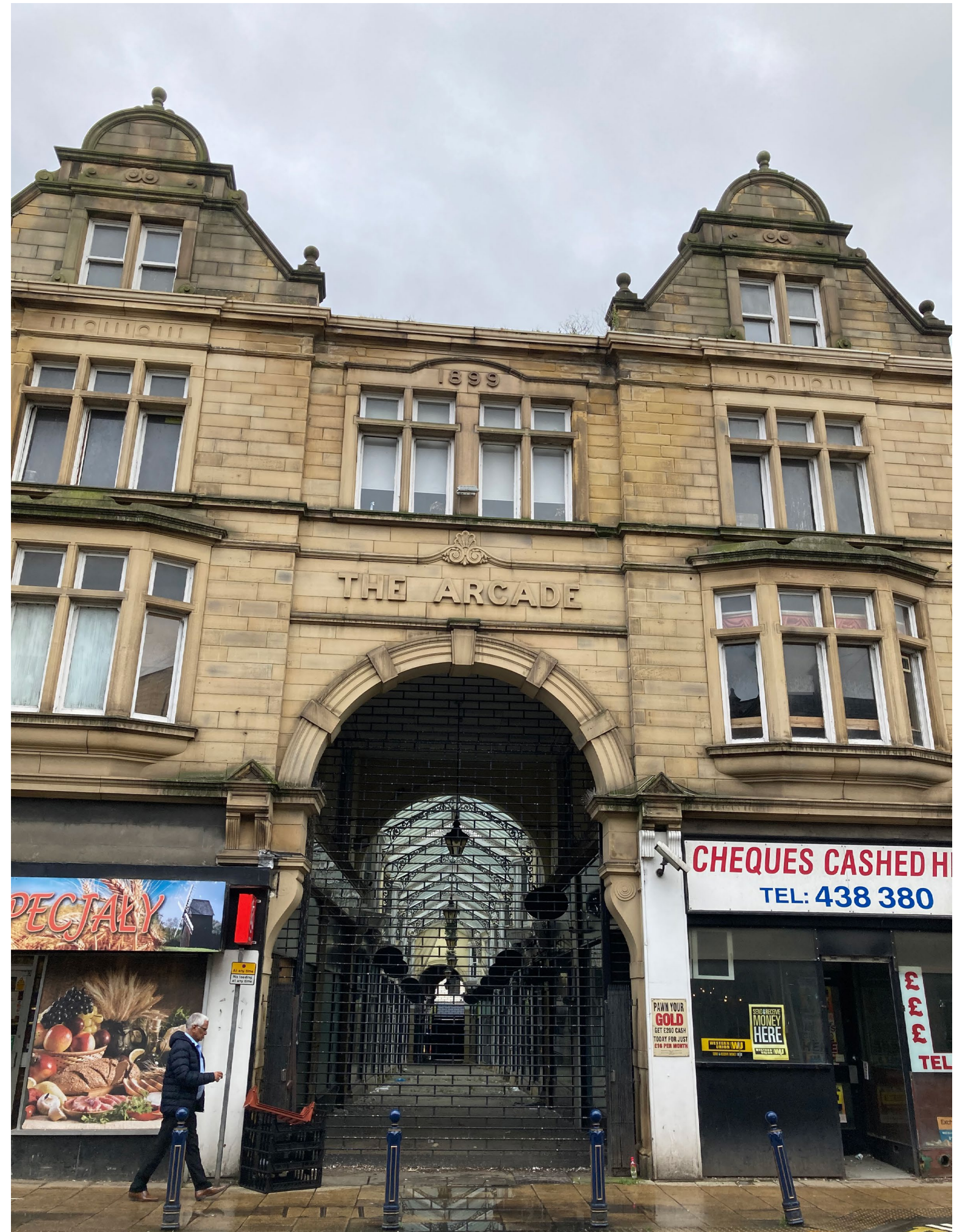
Figure 2.2.4 The Arcade Corporation Street façade (BDP 2021)
