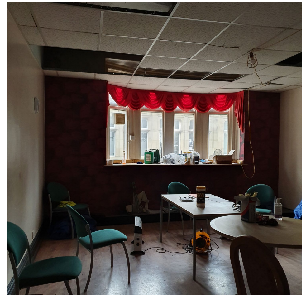
Figures 6.10.19 and 6.10.20 Site photographs of Corporation Street Levels 0&1 (BDP 2021)
