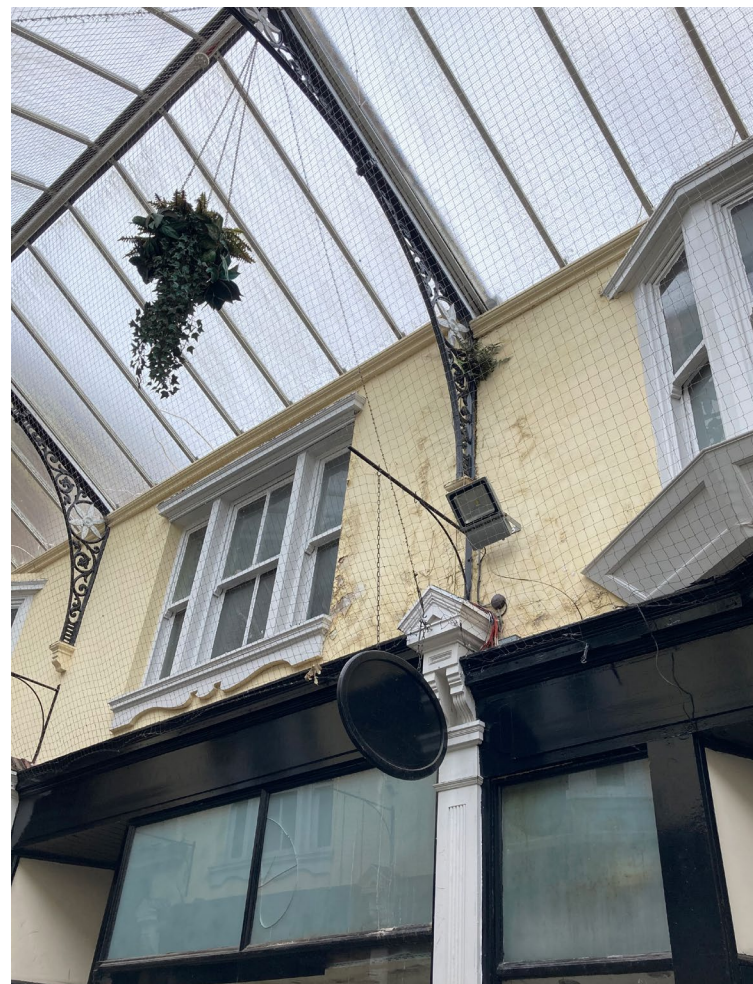
Figure 2.2.8 Cast iron trusses and decorative pilasters (BDP 2020)
