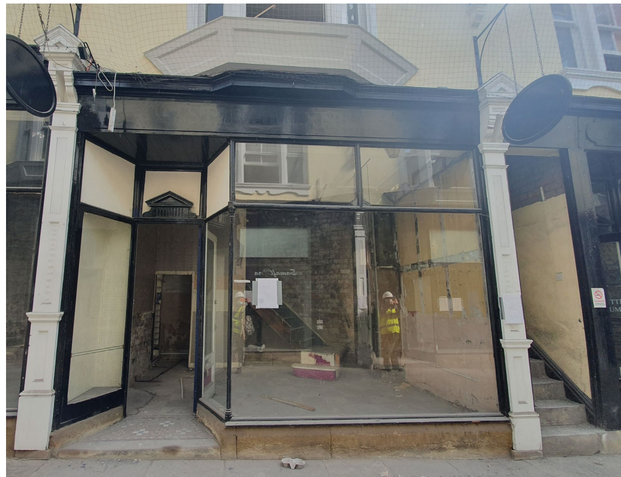
Figure 2.3.3 Arcade shop front with traditional details intact (BDP 2021)
