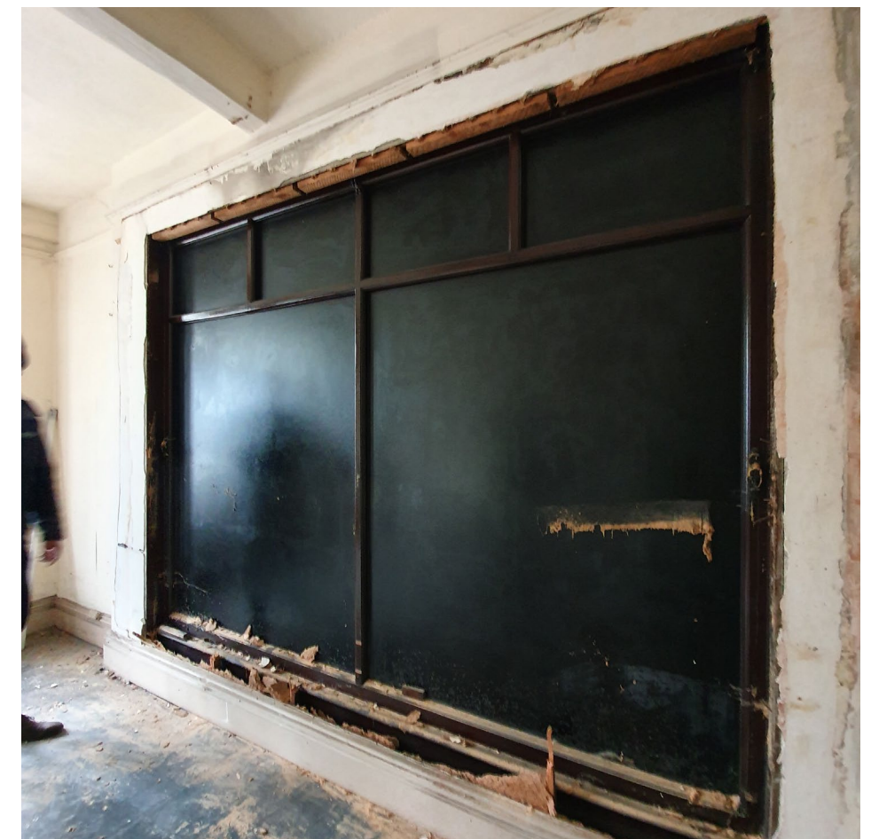
Figures 6.10.22 and 6.10.23 Site photographs of Market Place Level 1 (BDP 2021)
