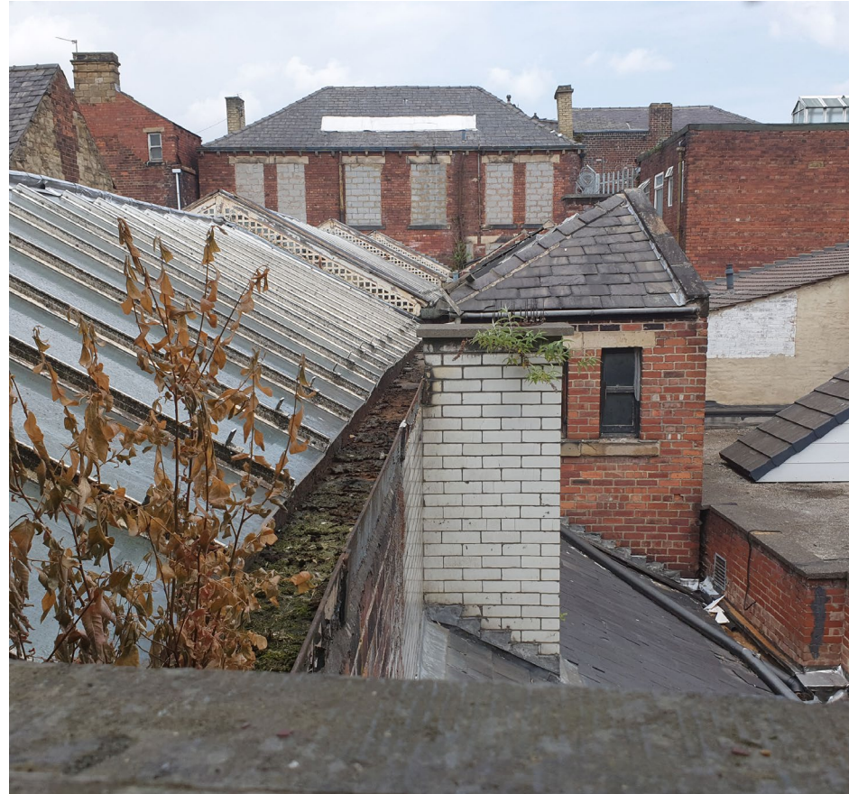
Figure 5.6.3 View of existing monopitch roofs from inside Market Place
