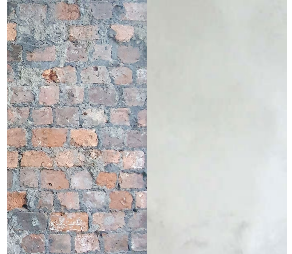
Wall finishes- Brick / lime plaster
