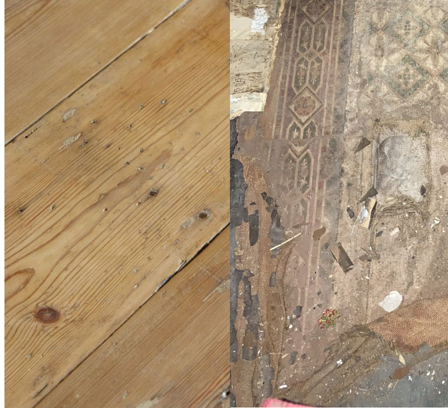
Floor finishes - Timber boards / restored early finishes
