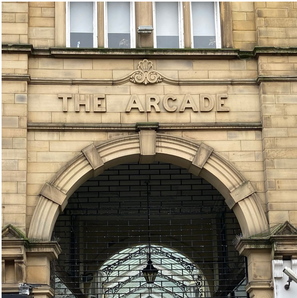
Historic fabric including masonry and metalwork with fine architectural detailing will be carefully conserved, refurbished and restored.
