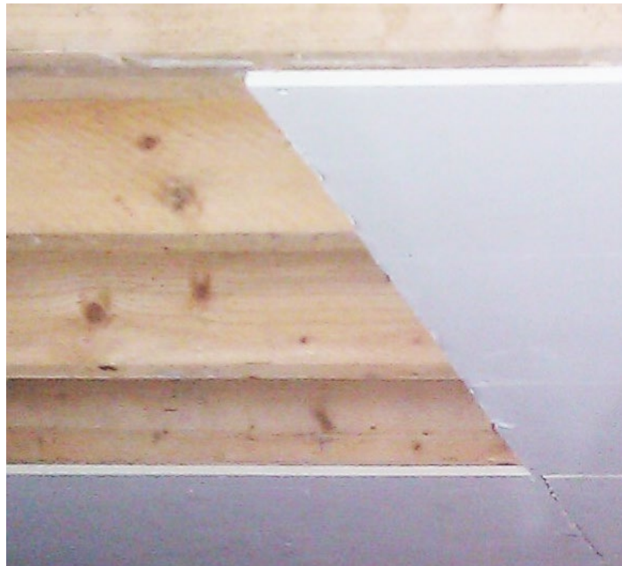
Ceiling finishes - Plasterboard
