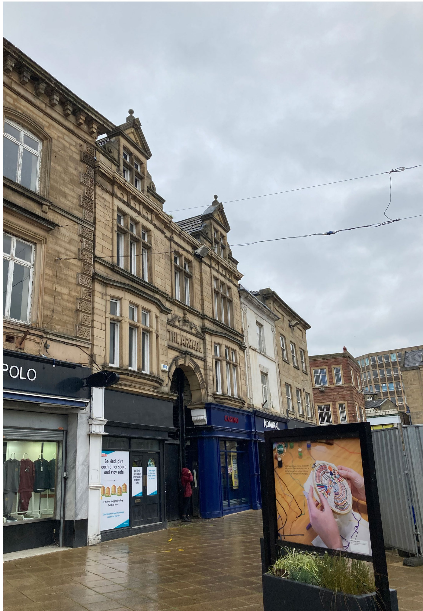
Figure 2.2.3 The Arcade Market Place façade (BDP 2021)
