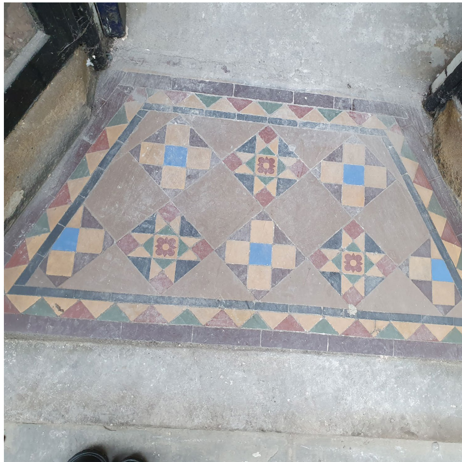
The decorative tiled thresholds that are part of the Dewsbury mosaic of visual interest are to be restored, and where lost, reinstated.
