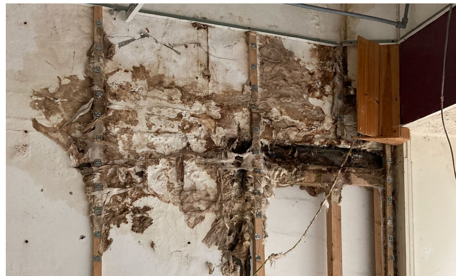
Figure 2.4.3 Incidences of dry rot (BDP 2020)
