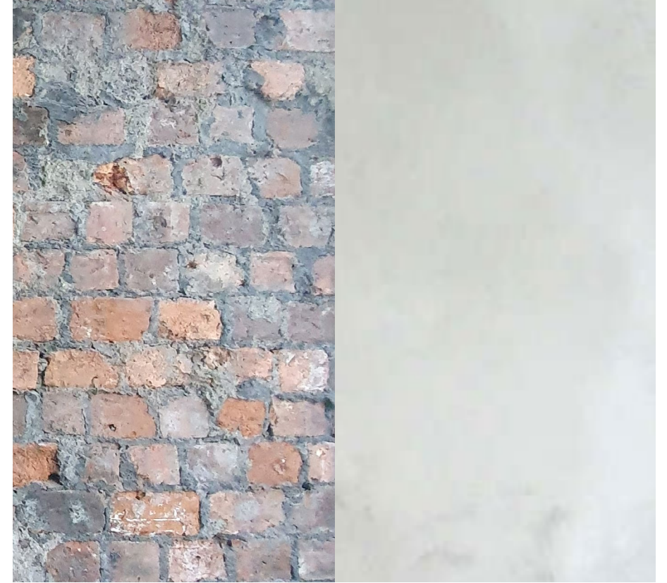
Wall finishes - Brick / lime plaster
