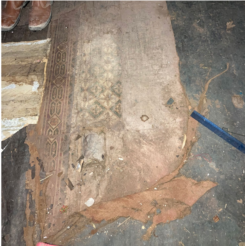
Concealed decorative floor finishes and internal glazed elements are to be retained and revealed where consistent with the new uses.
