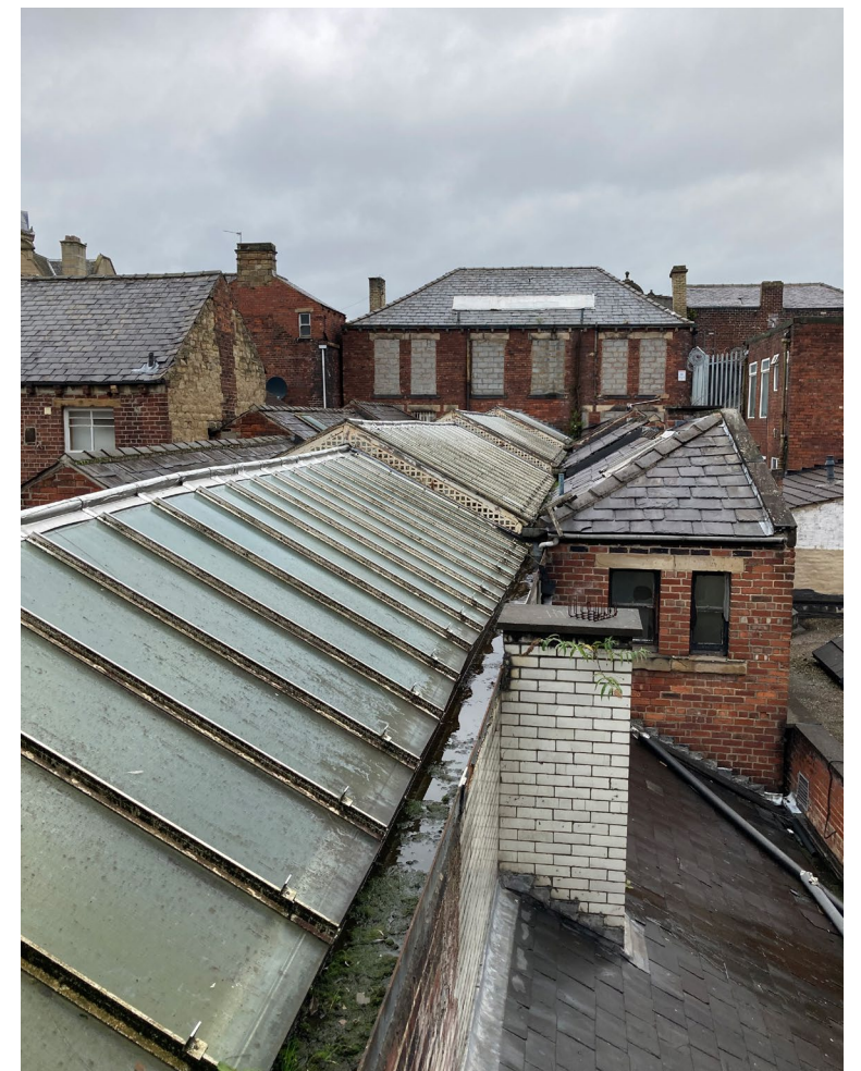
Figure 2.2.9 The central glazed roof (BDP 2020)
