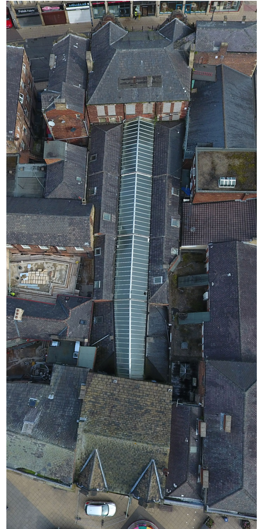
Figure 6.10.10 Aerial Drone Image (Watts roof survey 2021)
