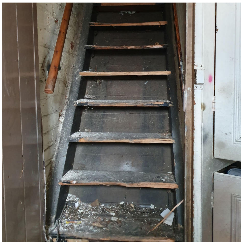
Figures 6.10.24 and 6.10.25 Site photographs of Market Place Level 2 (BDP 2021)
