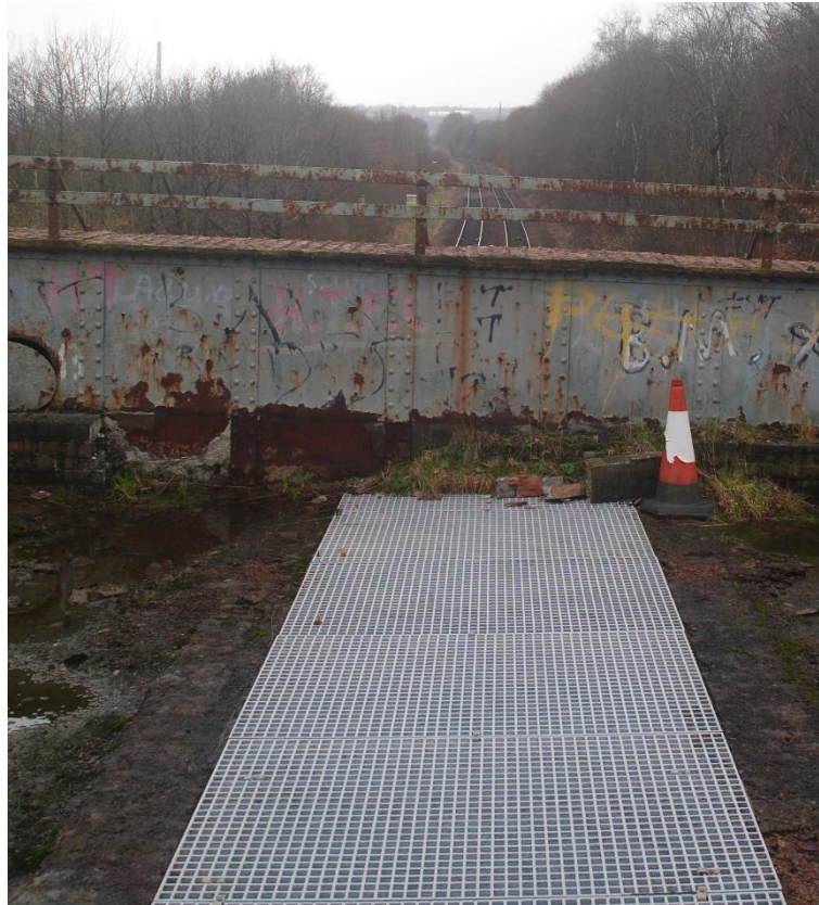
Plate A-2 - Western section of overbridge deck, viewed from east, from walkway.
