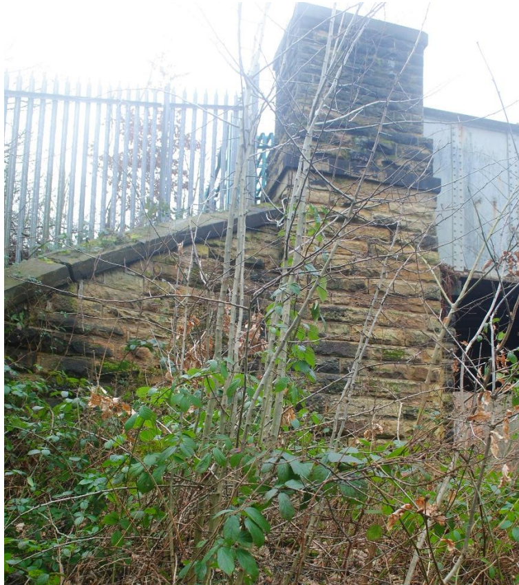
Plate A-5 - Southern abutment of overbridge, viewed from north-east.
