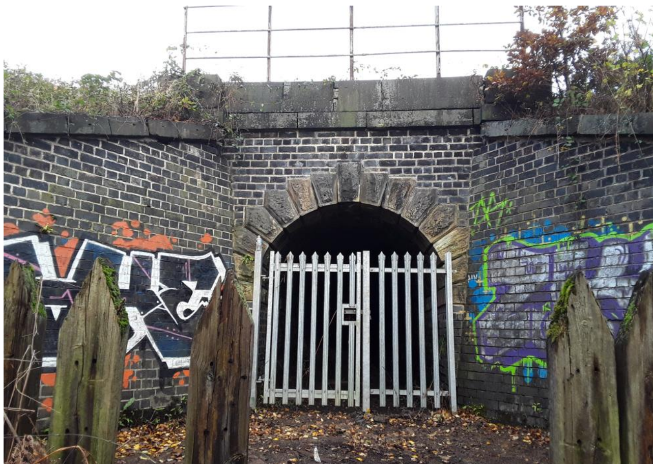
Insert 4-4 Peels Pit Underbridge (MVL 3/100) – southern elevation.
