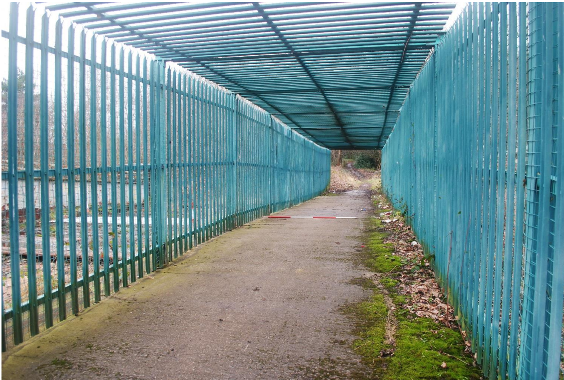
Plate 5-4 - General view of walkway over bridge deck, from south-east.
