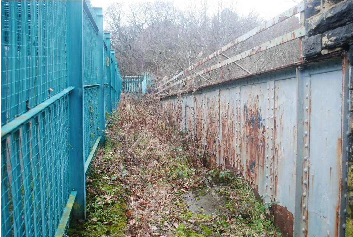
Plate 5-6 - Northern parapet of bridge, viewed from south.
