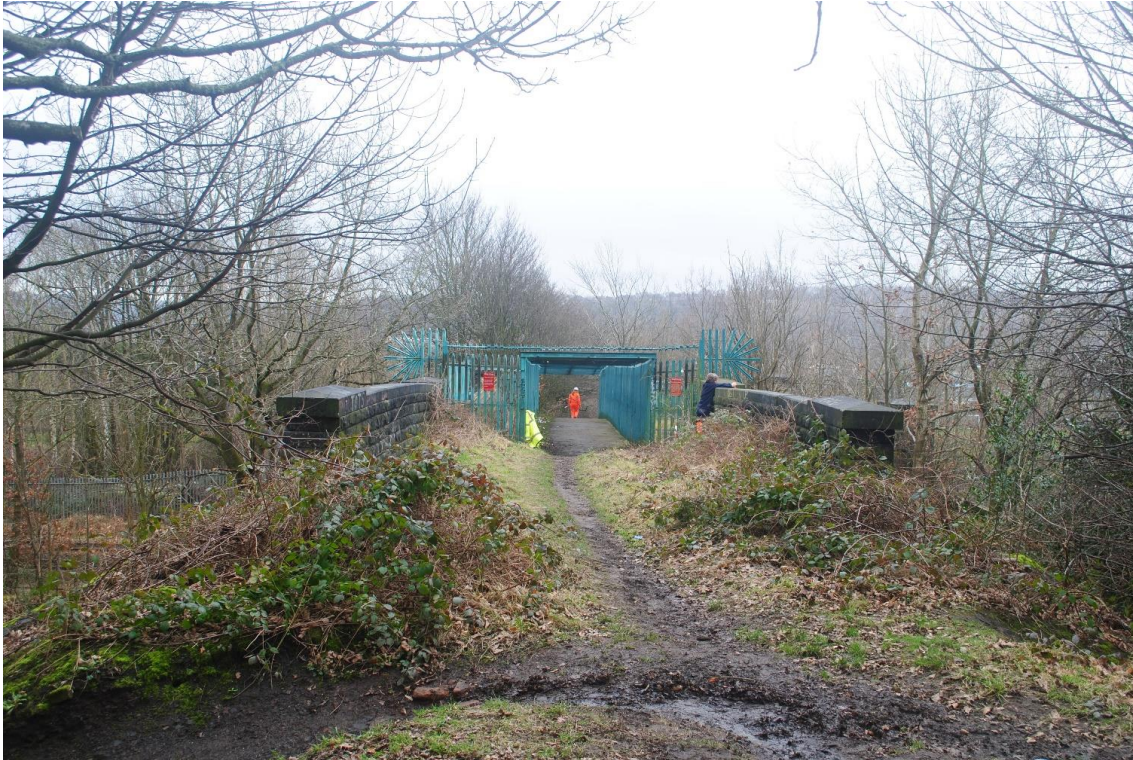
Plate 5-9 - Northern approach to overbridge, viewed from north. Note the former Midland Railway overbridge in the foreground.
