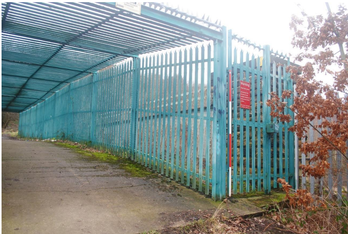
Plate 5-3 - General view of northern side of bridge deck, from south-west.
