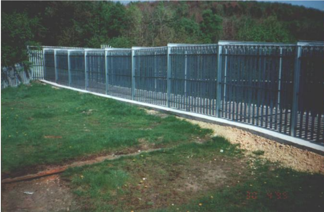
Plate 4-9 - View north-east across deck of Fieldhouse Overbridge (MVL3/98) showing addition of new walkway and fencing (Railtrack Inspection Report, April/May 1999) 17 .
