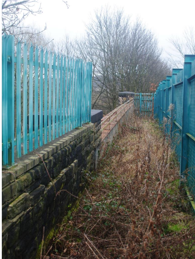
Plate A-4 - Eastern section of overbridge deck, viewed from north.
