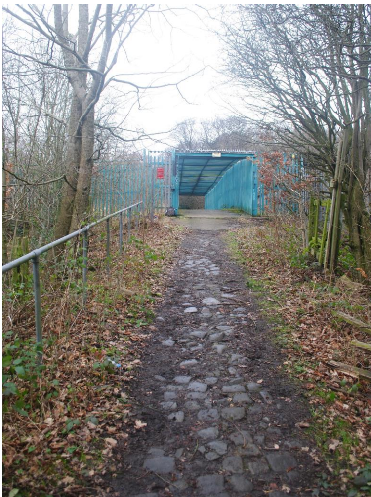
Plate 5-8 - Southern approach to overbridge.
