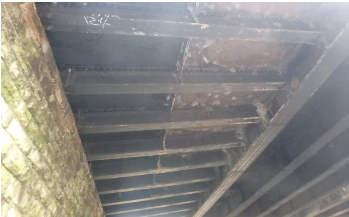
Plate 5-7 - General view of underside of bridge deck from south-eastern corner of abutment, showing main cross girders (right) and longitudinal girders at southernmost end of span (left) (Network Rail Inspection Report, November 2020).
