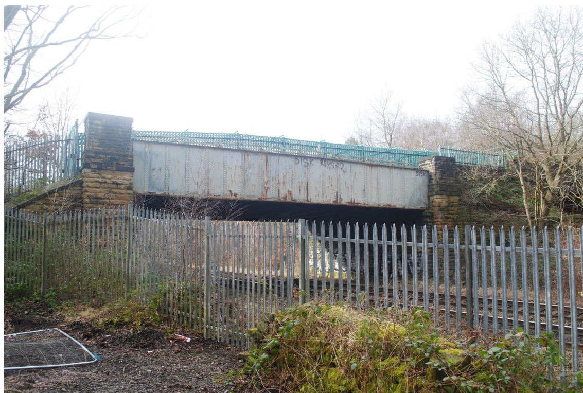
Plate 5-1 - Fieldhouse Overbridge (MVL3/98), general view of eastern elevation. Note the incline in the palisade fencing across the structure from left to right (south to north), evidencing the incline of the ground level over the bridge.
