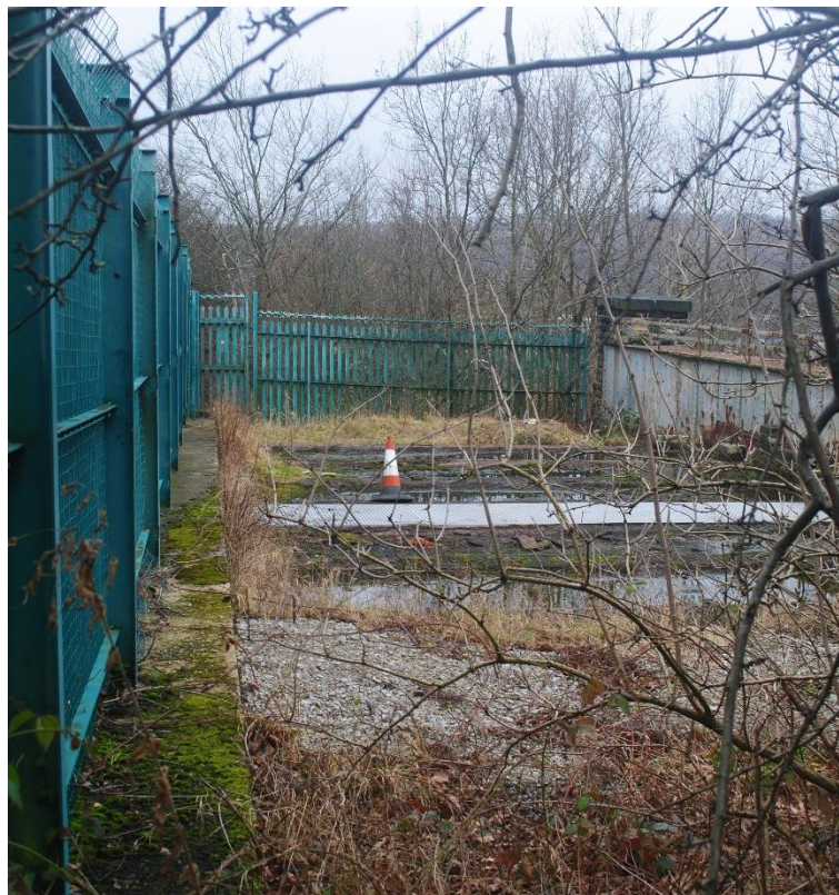
Plate A-3 - Western section of overbridge deck, viewed from north.
