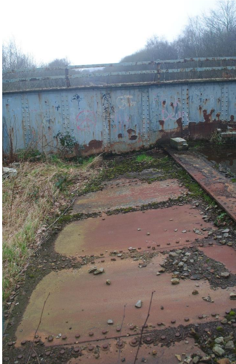
Plate A-1 - Western section of overbridge deck, viewed from east, from walkway.
