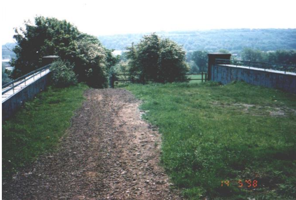
Plate 4-8 - View south across deck of Fieldhouse Overbridge (MVL3/98) prior to addition of fencing and caged walkway (Railtrack Inspection Report, May 1998) 16 .
