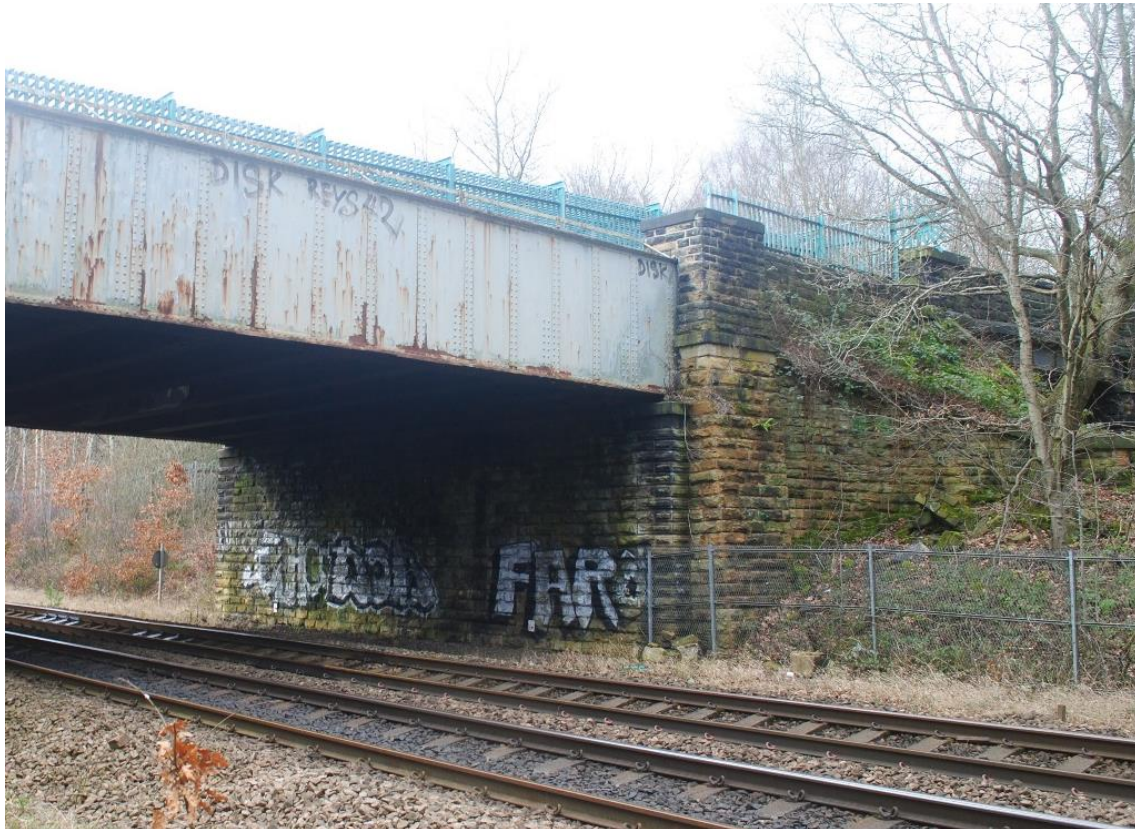
Plate 5-2 - Northern abutment of overbridge.
