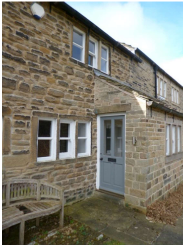
It is proposed to replace these doors with a stronger timber doors with heritage double safety glazed units in the same style with suitable security ironmongery
