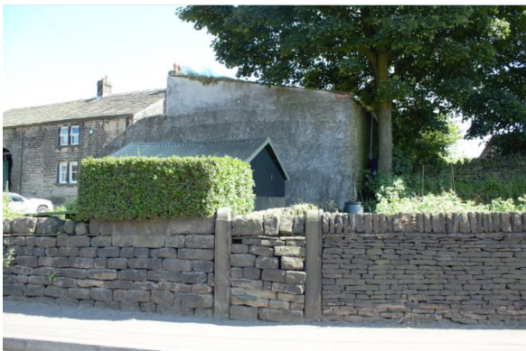
Figure 21: View of historic stone gateposts facing Butts Road
