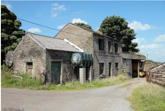
Figure 19: Former Yew Tree Farm farmhouse (derelict)
