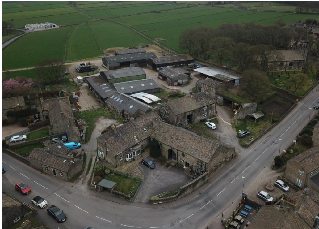
Figure 2: Aerial photograph looking south, showing the existing site
