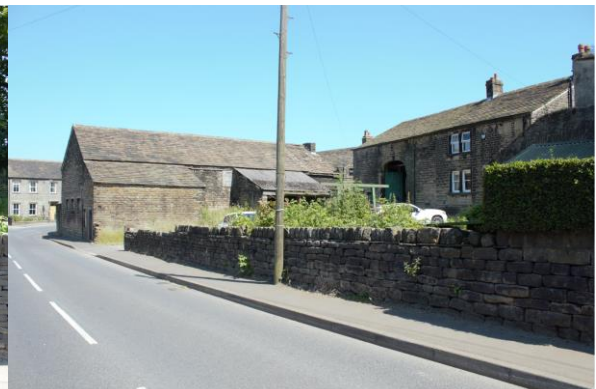
Figure 22: View of historic boundary wall along Butts Road
