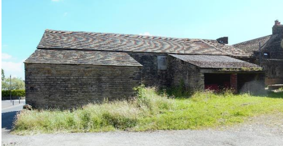
Figure 15: Lean-to extensions to principal (former Manor Farm) barn
