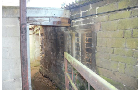
Figure 12: Blocked mullioned window on West side of former dairy
