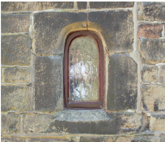
Figure 17: Small arched window on 55 The Village
