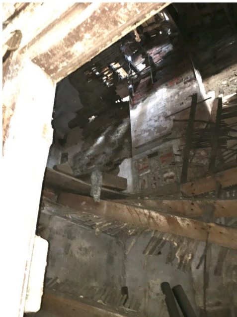
Collapsed first floor and ceiling structures
