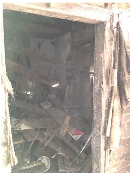
Collapsed first floor and ceiling structures
