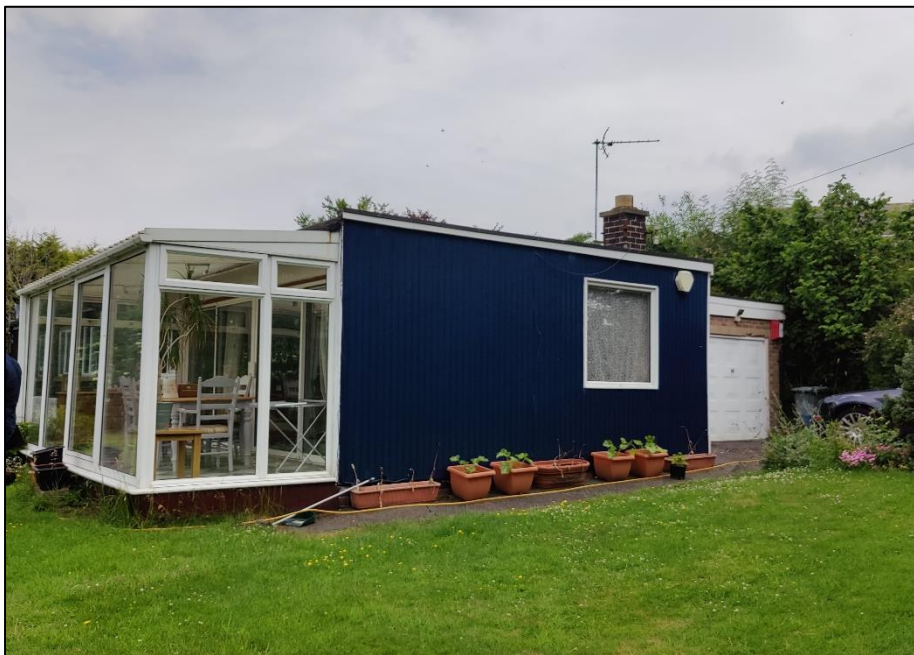
Photograph showing existing front (western) elevation
