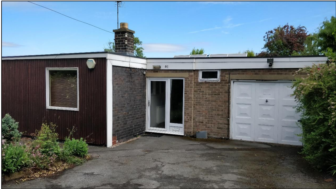
1970's extension on the right (lighter brick colour – not same height as main house)
