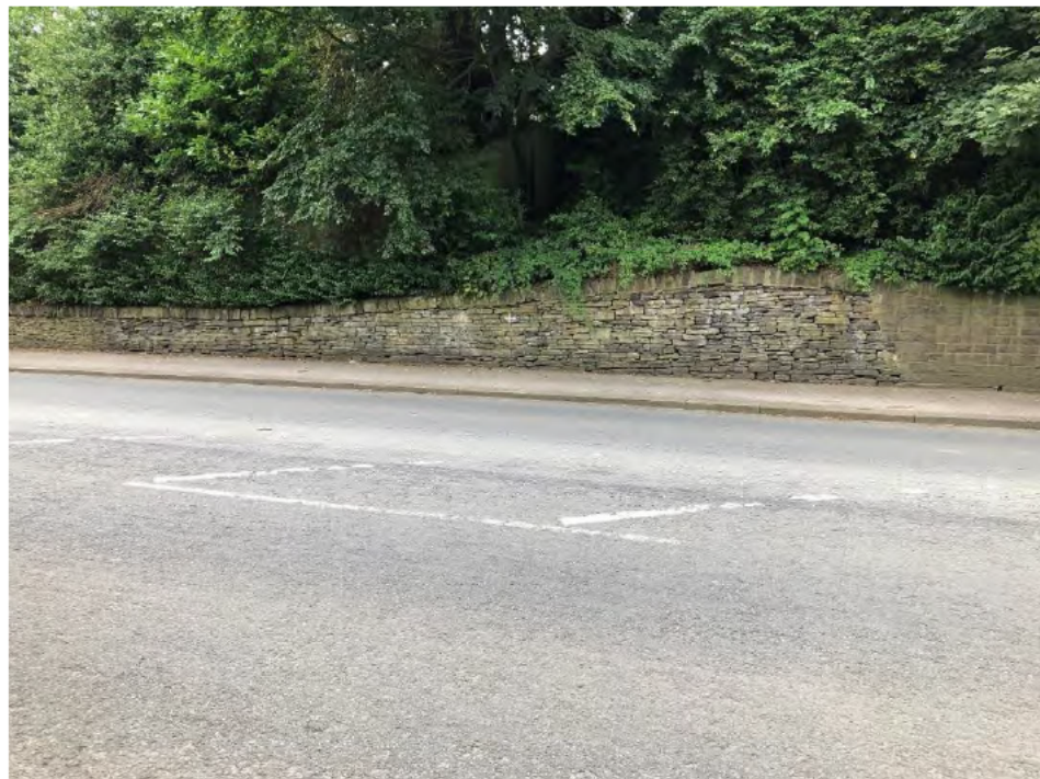
Image 7 View of north-western end of wall
