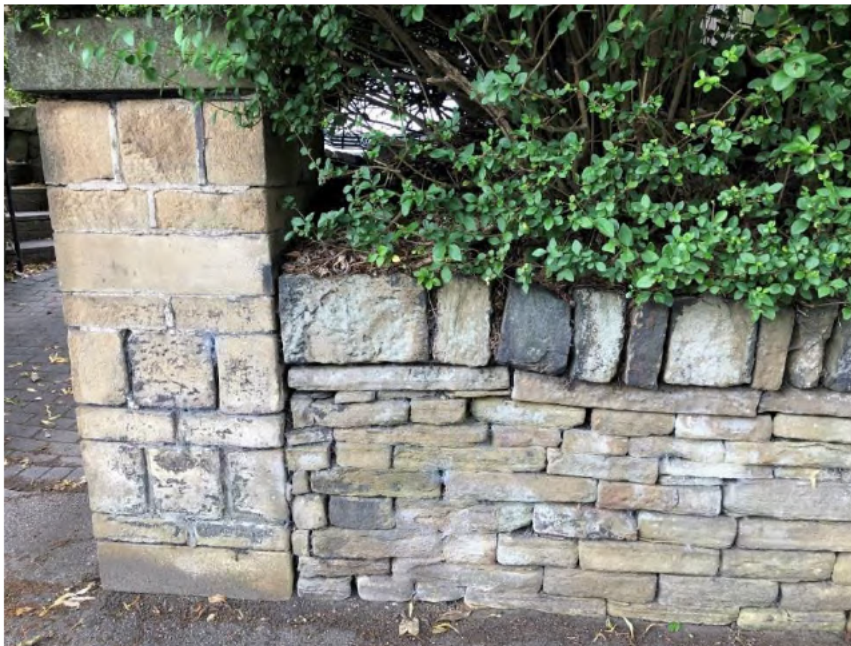
Image 5 North-western gate pier and adjacent wall
