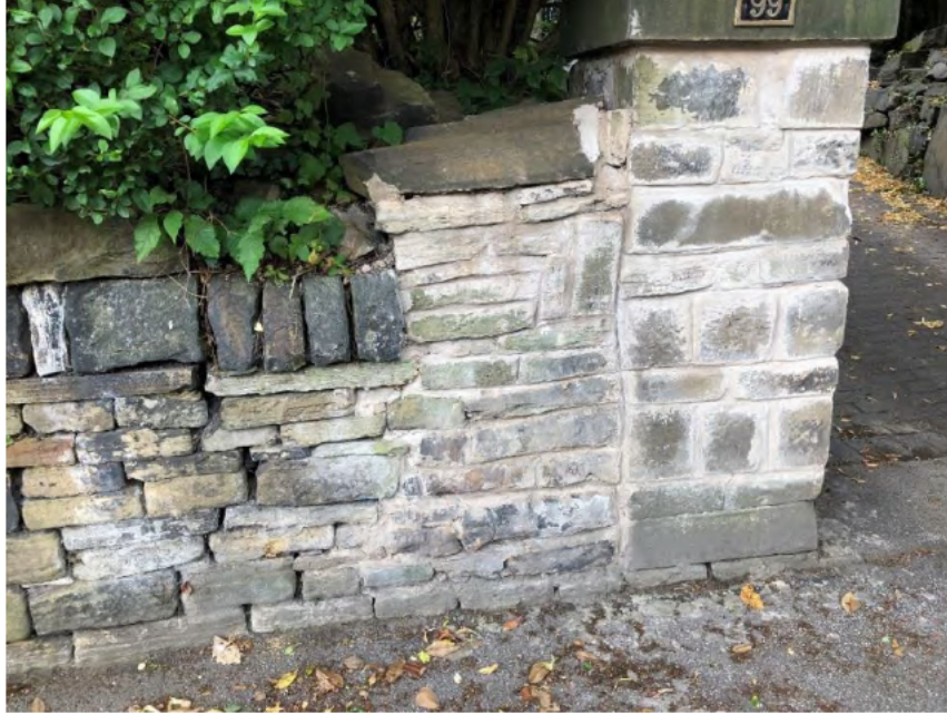
Image 4 South-eastern gate pier and adjacent wall
