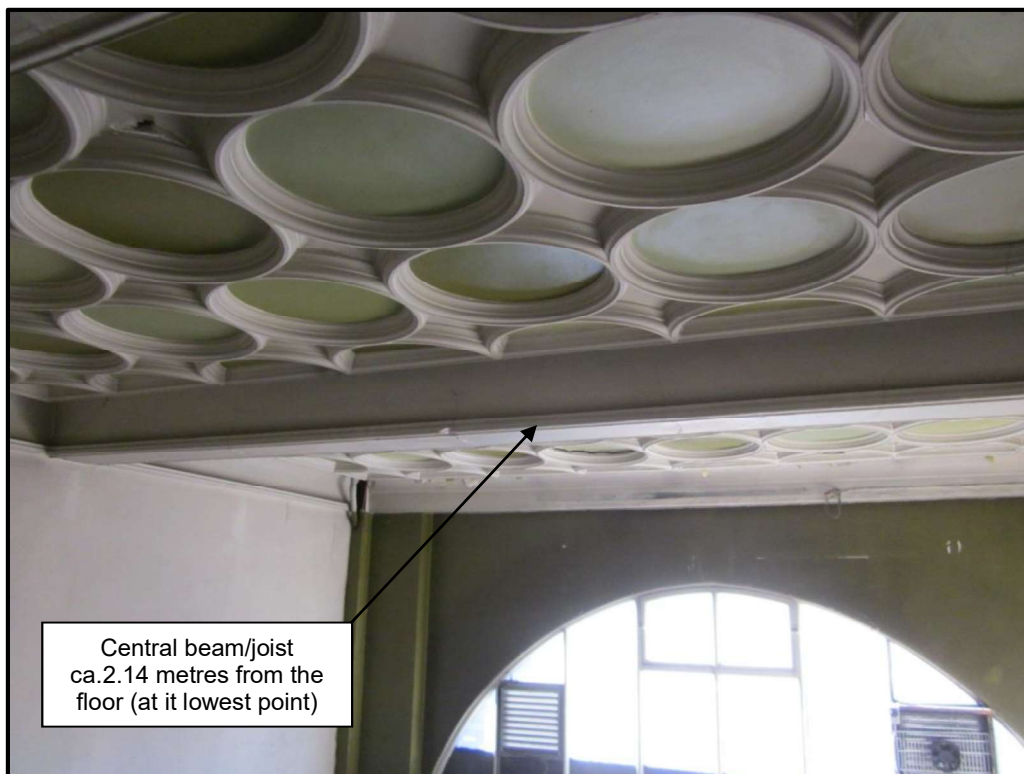
Photograph 4. Existing ceiling structure, 24 Westgate
