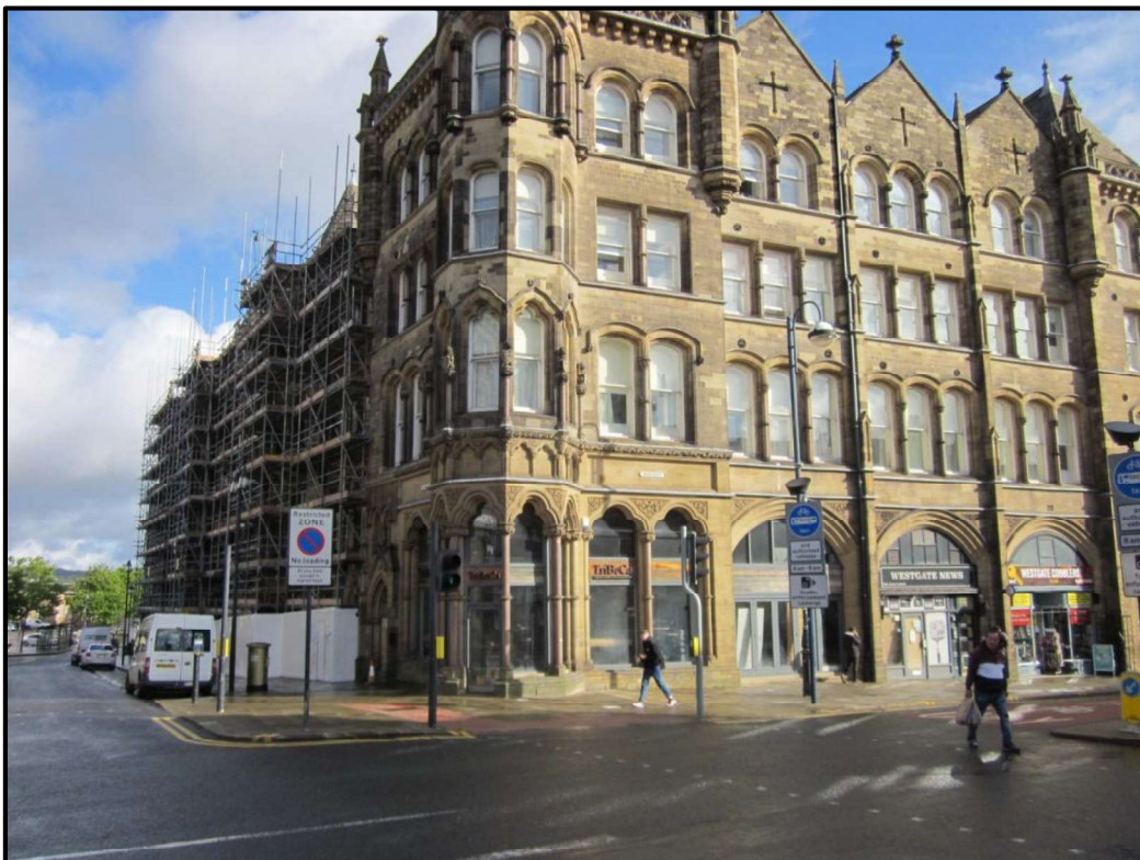
Photograph 3. Residential flats directly above the commercial premises on Westgate
