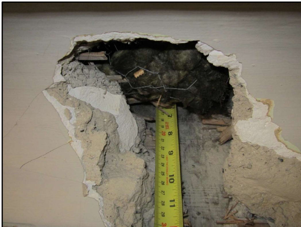
Photograph 5. Existing floor construction, 24 Westgate
