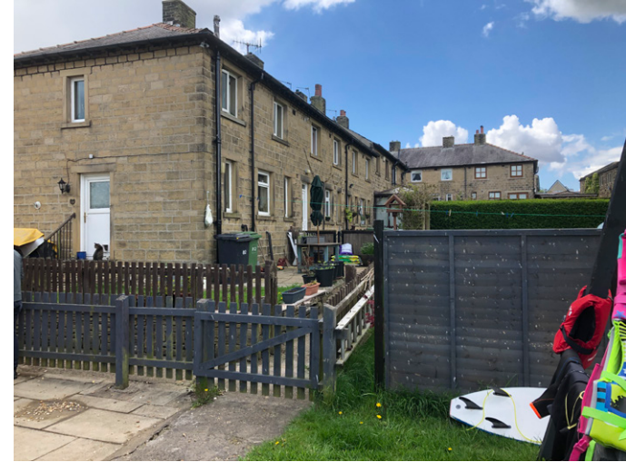
SIDE / REAR VIEW OF NO. 82
