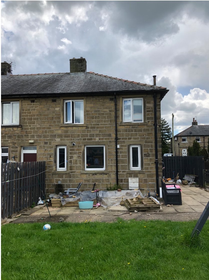
REAR ELEVATION (NO. 78 TO LEFT OF PICTURE)
