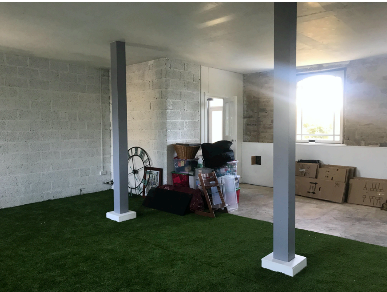
internal view from point A
