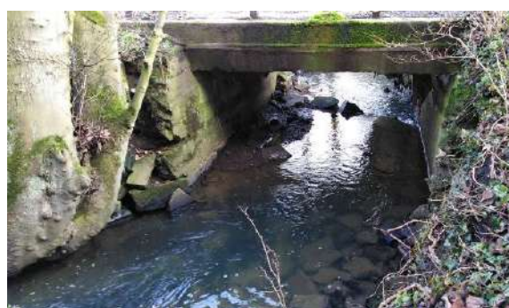
Photograph 8: Park Gate Dike running beneath the access track (looking east)
