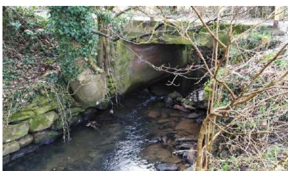
Photograph 7: Park Gate Dike running beneath the access track (looking west)
