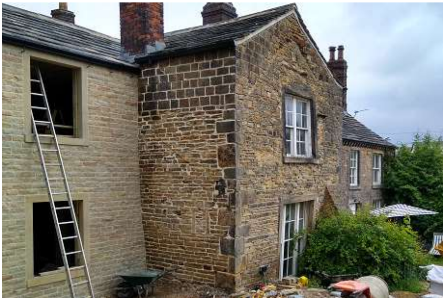
Photograph 1. Location of carved stone on SW corner
