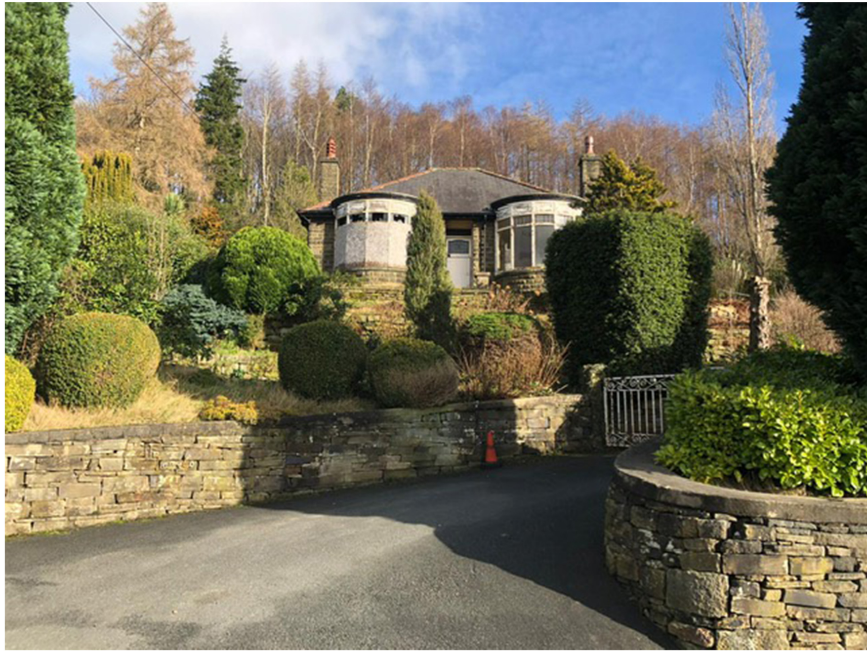
Existing view of The Laurels from Coldhill Lane
