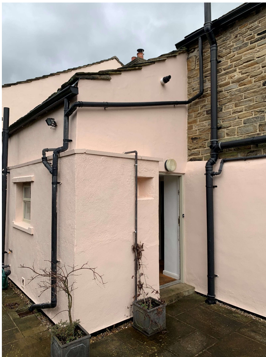
View from the patio area of the existing entrance door and continuation of the lean-to roof.
