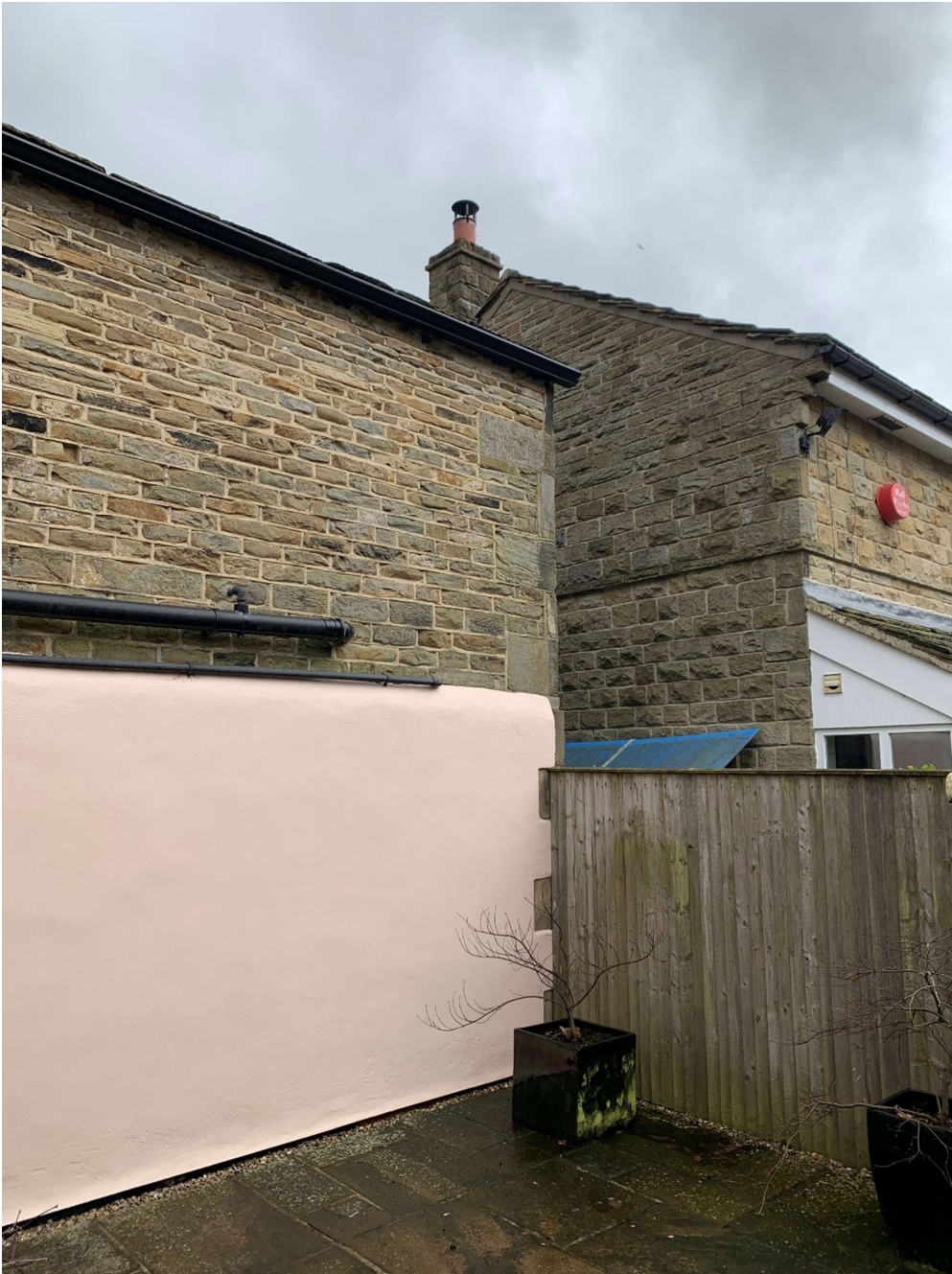
View from the patio of the extent of existing rendered wall to be removed (and waste pipes hidden). The modern property, Mollicar House, adjacent can be seen to the other side of the boundary fence.
