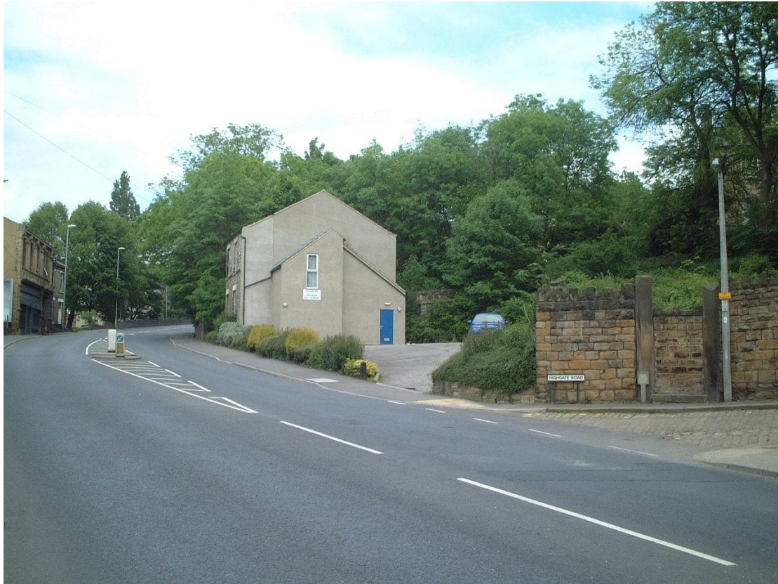
Photograph To Show South Elevation And Access To 30 Leeds Road.
