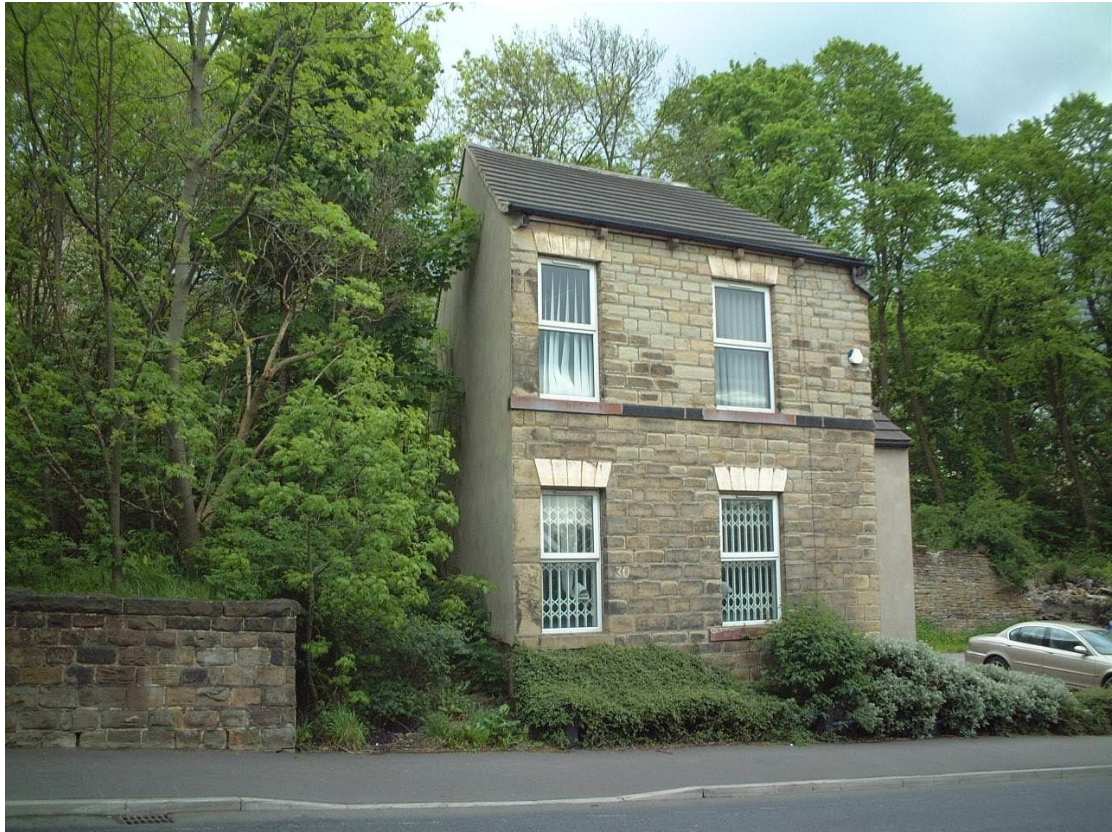
Photograph To Show North And West Elevation Of 30 Leeds Road.
