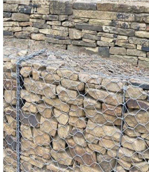
examples of retaining wall materials and designs using gabion baskets, or stone wall, or even a mix, and all will be landscaped
