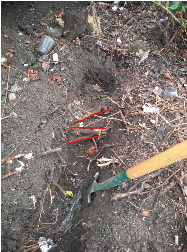
Trench for Tree 14 showing the position of three roots from the tree, together with roots from shrubs.
