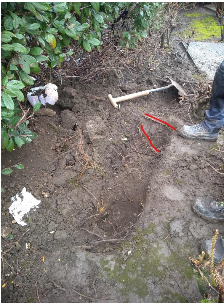
Trench for Tree 12 showing the position of two small diameter roots from the tree and lots of roots from shrubs.
