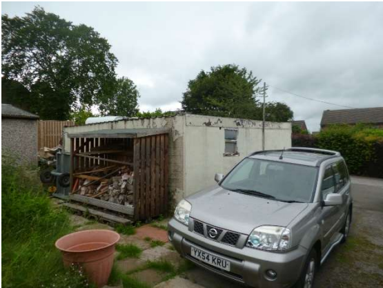
Rear of double garage to be demolished
