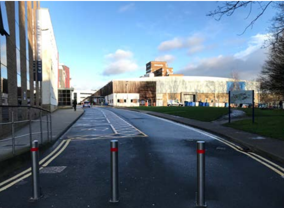
View of the site from the South, on the route into the Campus from the Barbara Hepworth building
