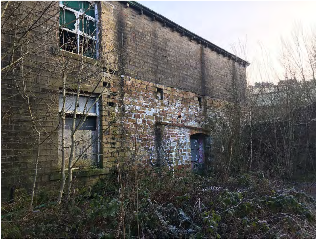
Photo 15. West elevation of building
