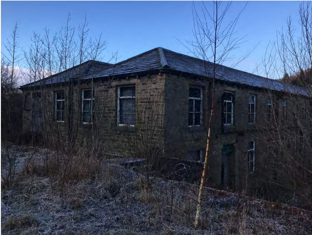
Photo 13. Looking north-west to building on the site
