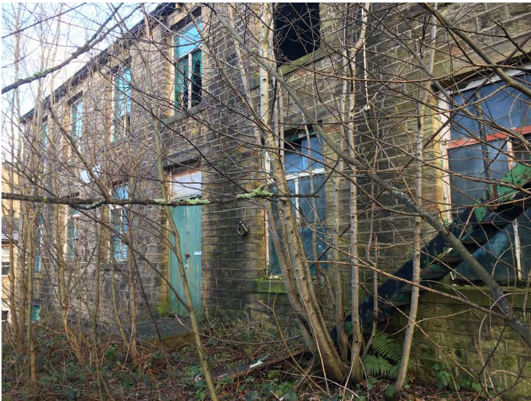
Photo 14. West elevation of building
