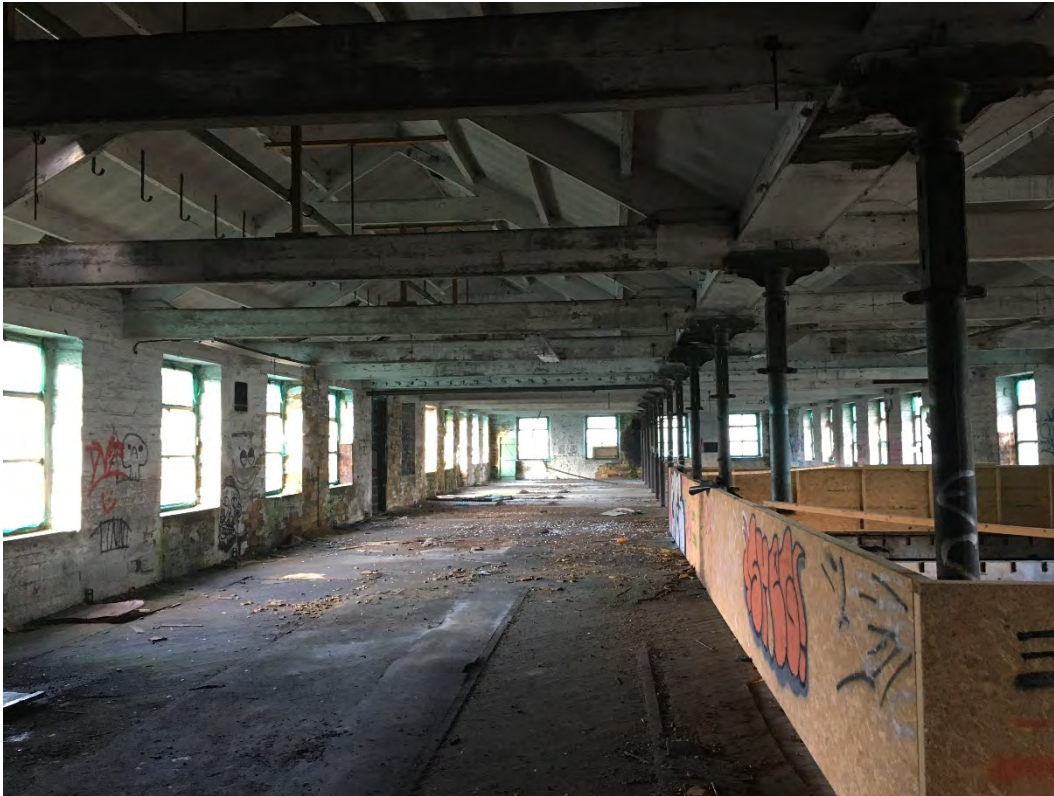
Photo 17. First floor within building
