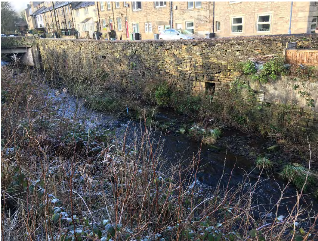
Photo 6. Looking west across River Holme in western part of the site
