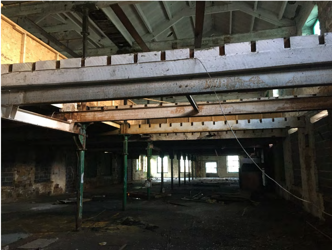
Photo 16. Looking north-west within ground floor of building
