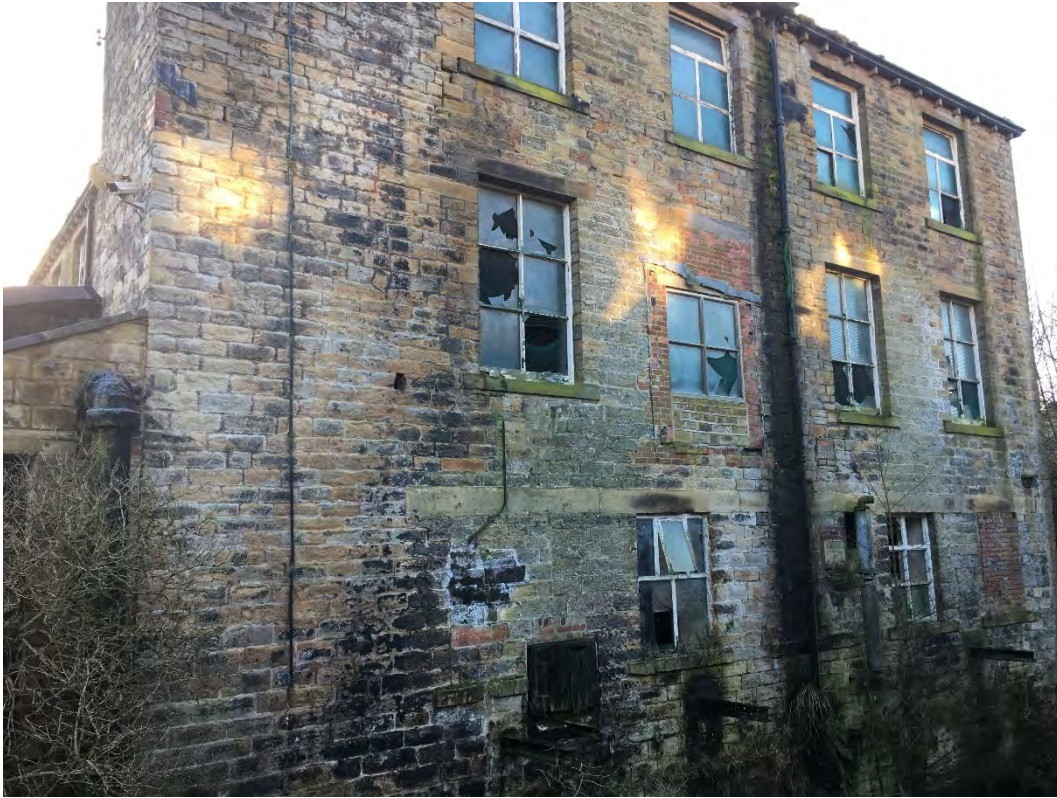
Photo 9. North-west elevation of building on the site
