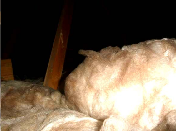
P8 Loft, thick layer of insulation
