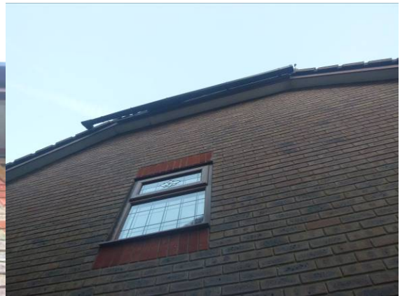
P4 NW gable, well-sealed
