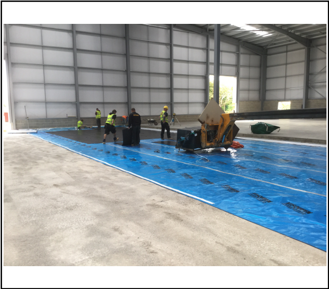
Photo 1 - Blinding being laid in sections
