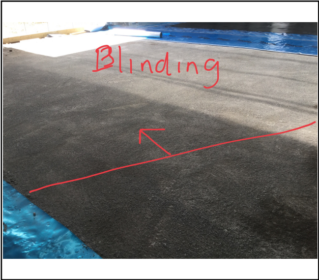
Photo 1 - Blinding being laid in sections
