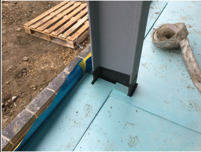
Stanchion prior to Membrane
