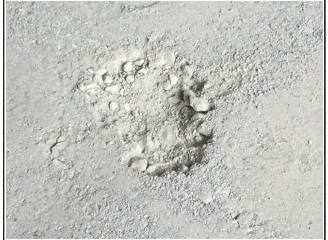
Sand Blinding Repair
