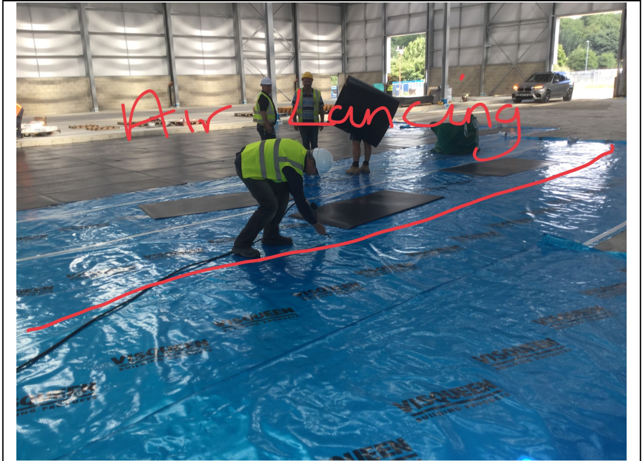
Photo showing Air Lancing being undertaken
